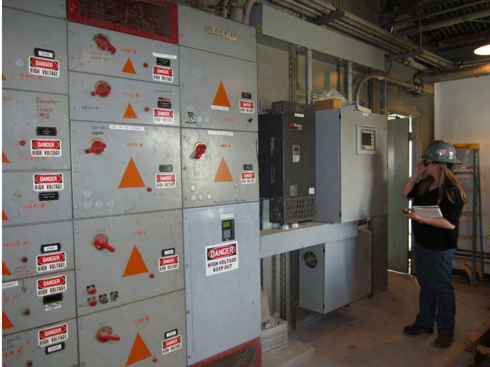
Gould electrical panel, variable frequency drive and PLC
