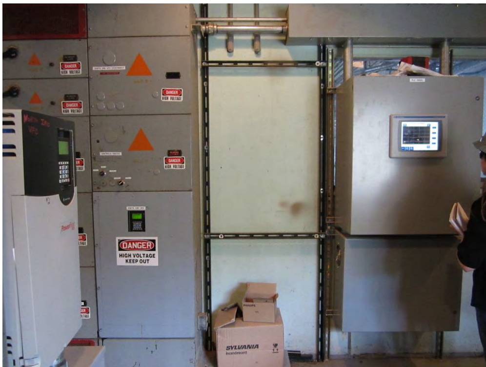
Dry Creek variable frequency drive, electrical panels and PLC
