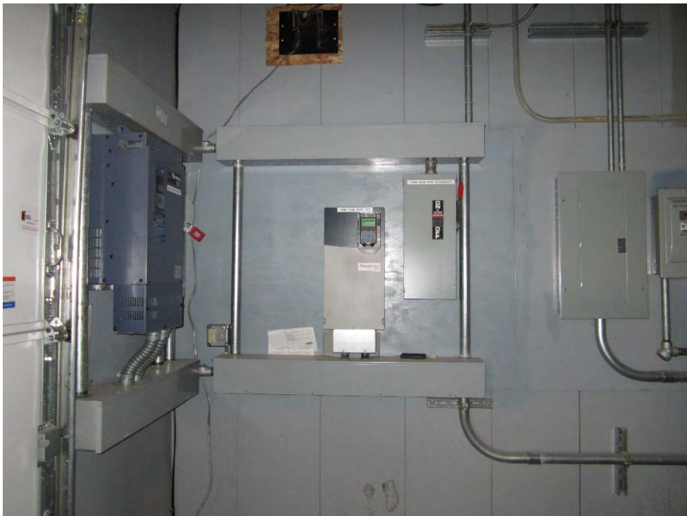
Oregon Basin tank gear pump variable frequency drive and shutdown
