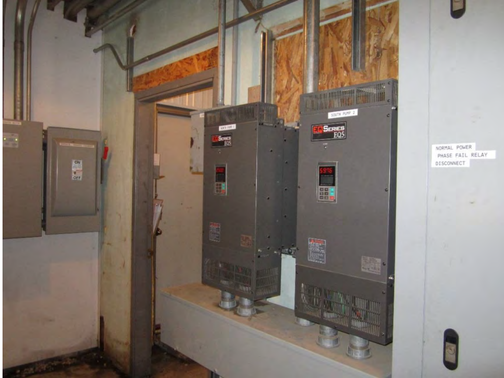
Fourbear pump variable frequency drives and shutdown
