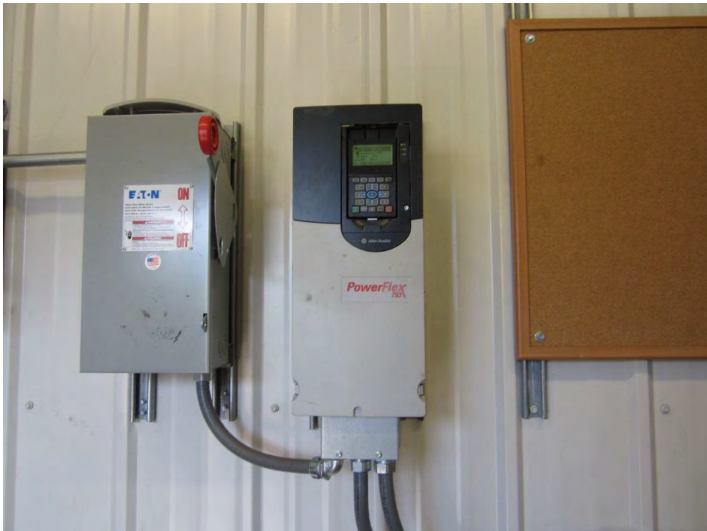
Battery #1 pump variable frequency drive and shutdown
