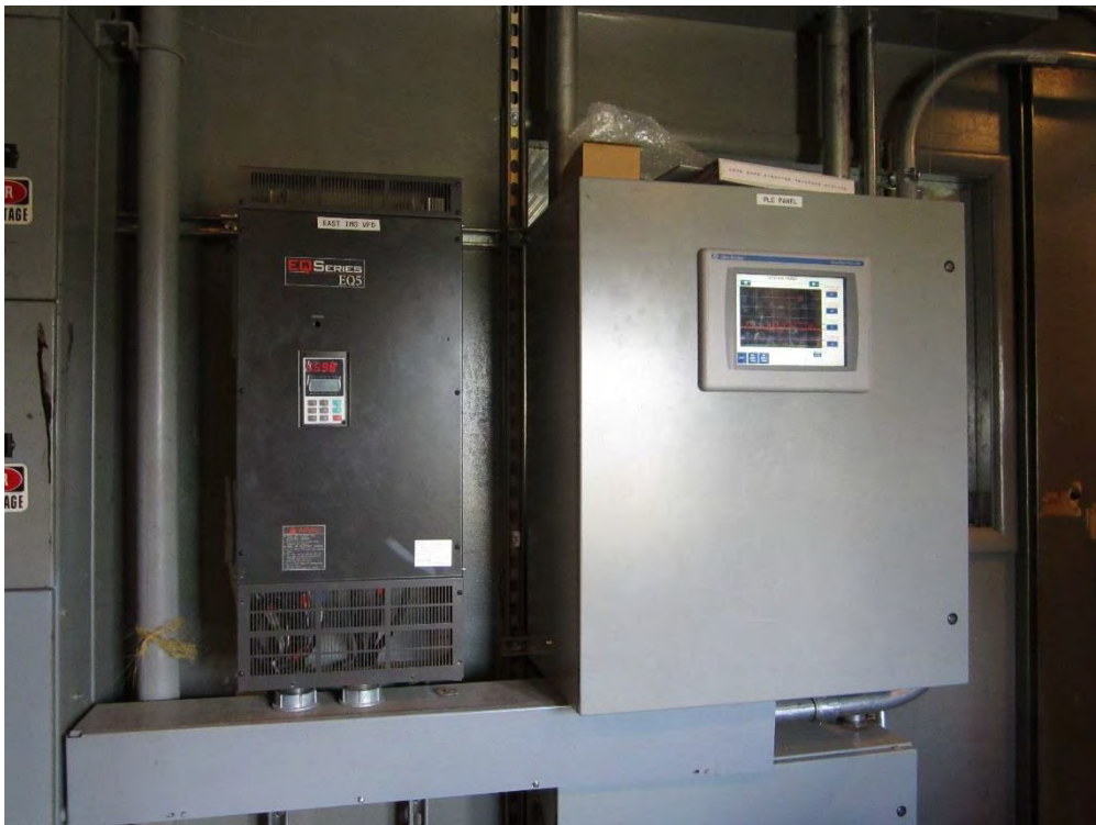
Gould pump variable frequency drive and PLC
