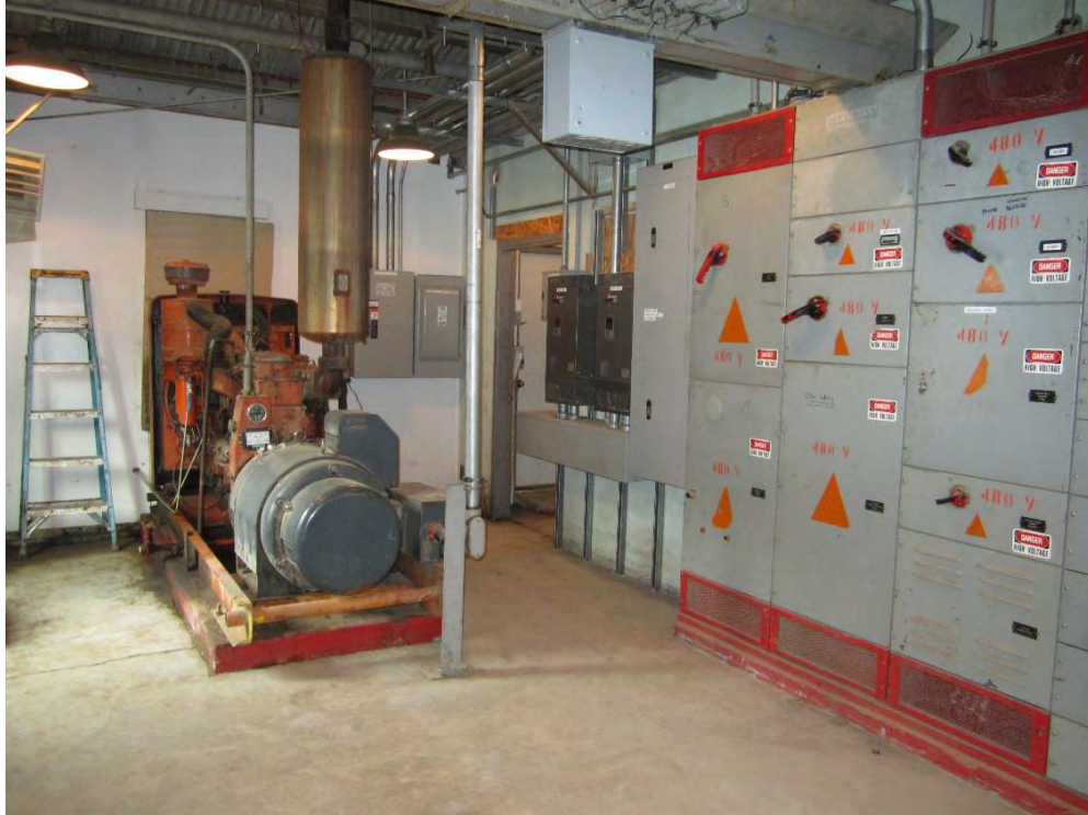
Fourbear electrical panel and pump variable frequency drives
