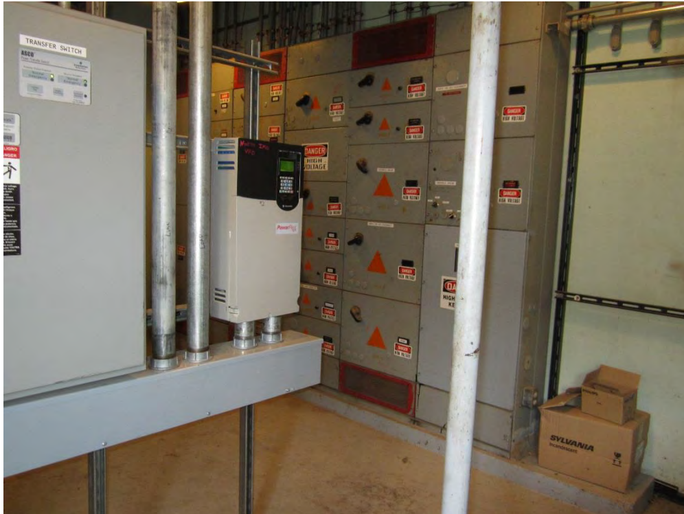
Dry Creek variable frequency drive and electrical panels
