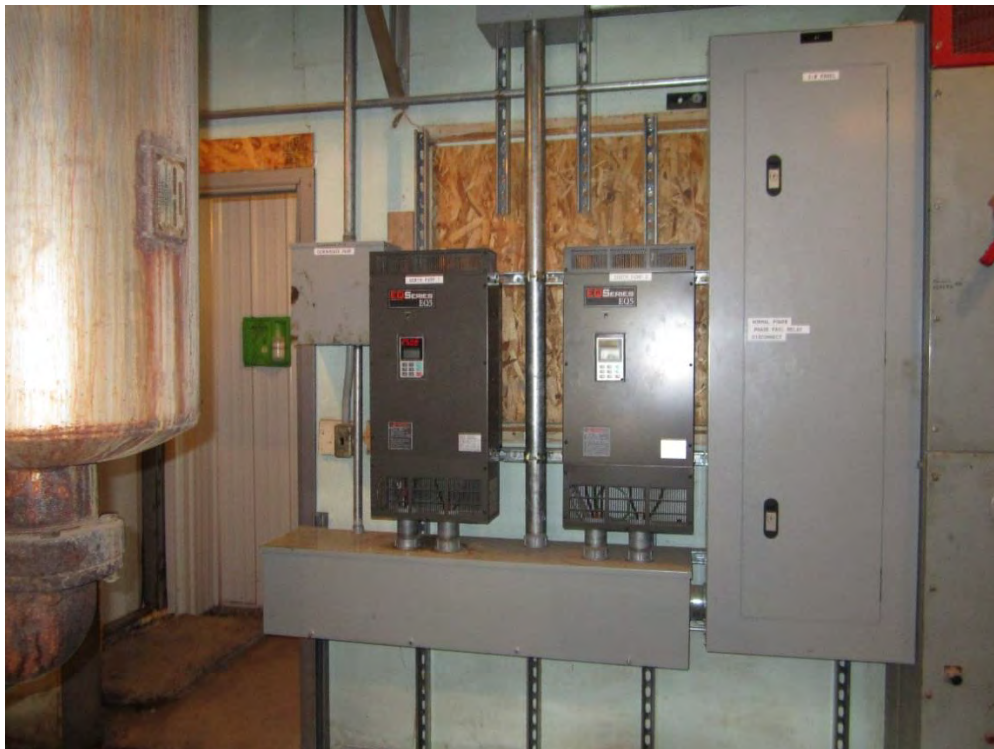
Fourbear pump variable frequency drives
