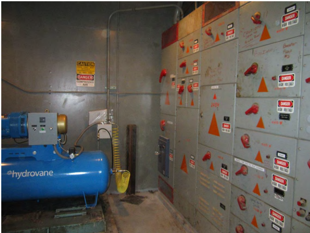
Gould electrical panel and setting
