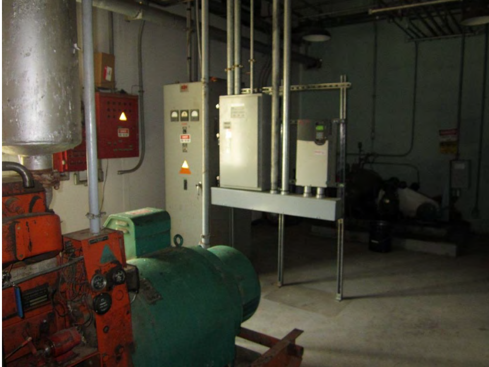
Dry Creek pump variable frequency drive
