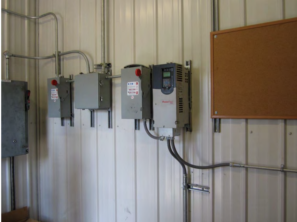
Battery #1 pump variable frequency drive and shutdown
