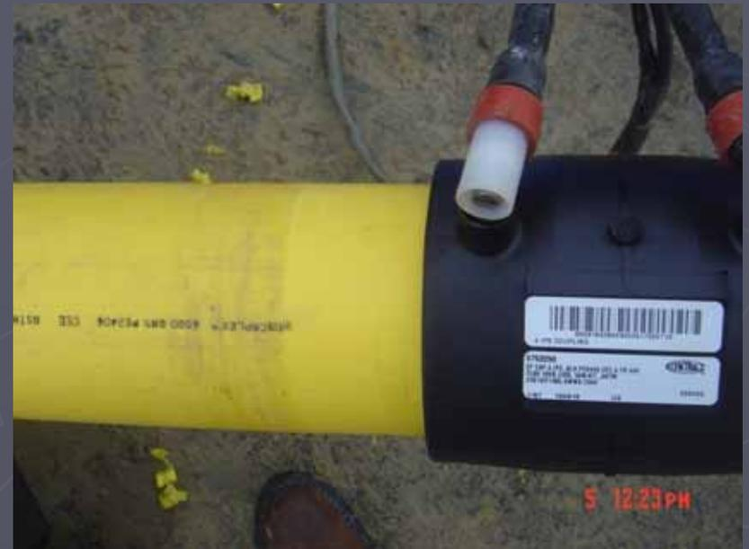
Another example of not marking the proper stab depth before performing an electrofusion.
