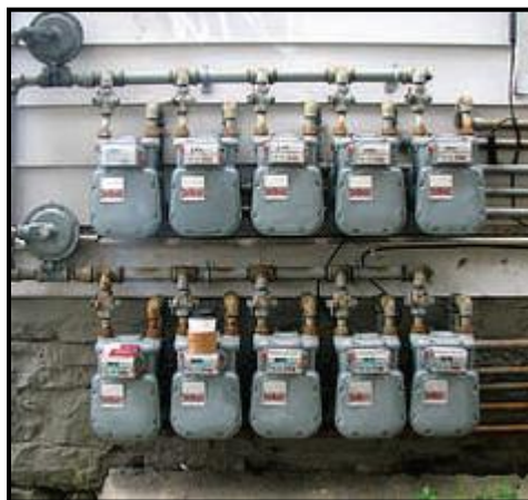
Figure 12 - Service through a Meter Manifold
