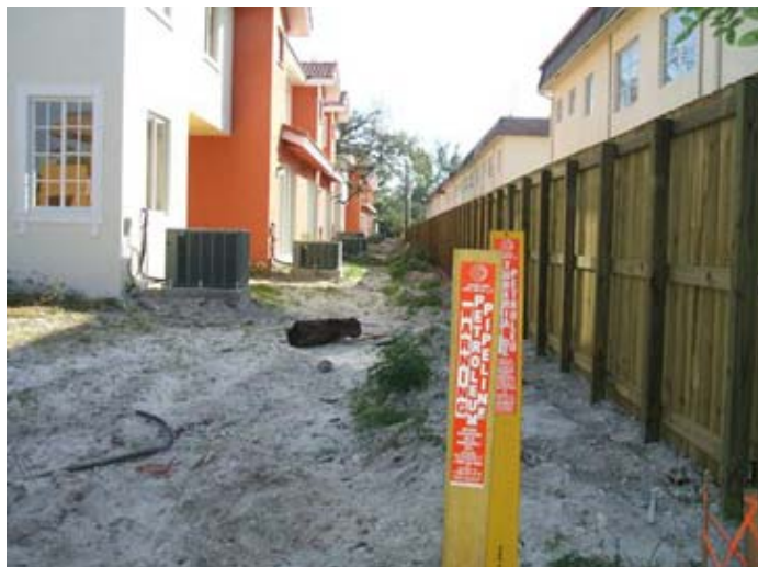
Figure 5.1 – Pipeline encroachment in residential development. http://www.apga.org/library/PHMSA%20notices/PIPA_Flier_Final.pdf
