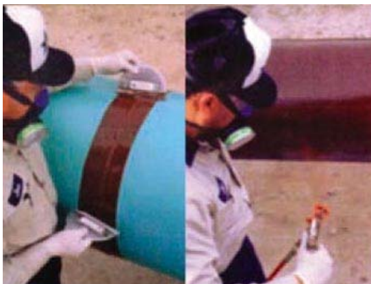
Figure 5.5 – Powercrete® pipeline coating application ( http://www.petropages.com/vendors/v19548.htm )
