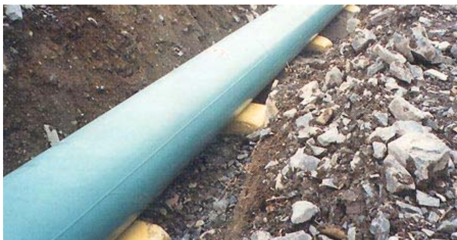
Figure 5.6 – Pipeline on Foam Supports ( http://www.pedero.com )
