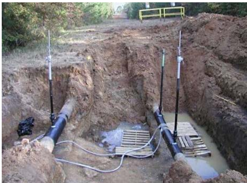
Figure 5.13 – Daylighted Pipeline Site (Courtesy: http://www.process.sensorsmaq.com )
