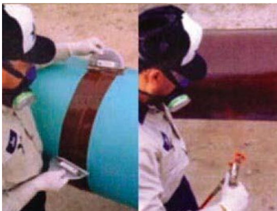
Figure 5.5 – Powercrete® pipeline coating application ( http://www.petropages.com/vendors/v19548.htm )
