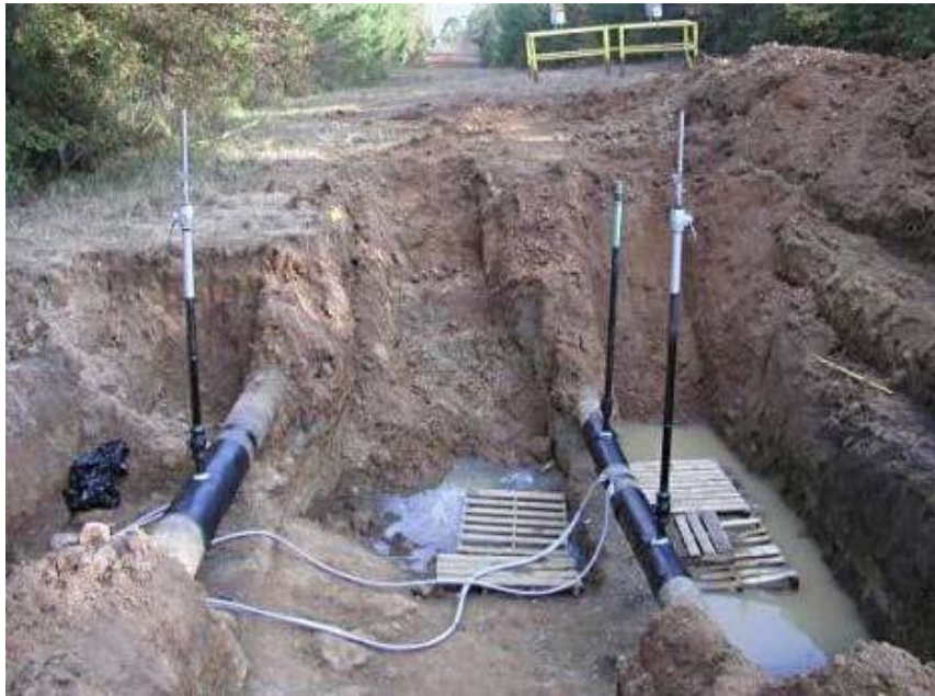
Figure 5.13 – Daylighted Pipeline Site (Courtesy: http://www.process.sensorsmag.com )
