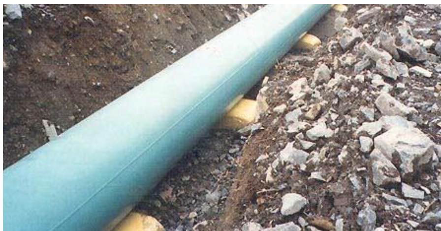
Figure 5.6 – Pipeline on Foam Supports ( http://www.pedero.com )
