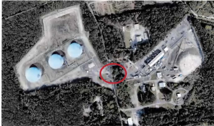
Overhead photographs of facility with Wilson Street pipe crossing circled in red
