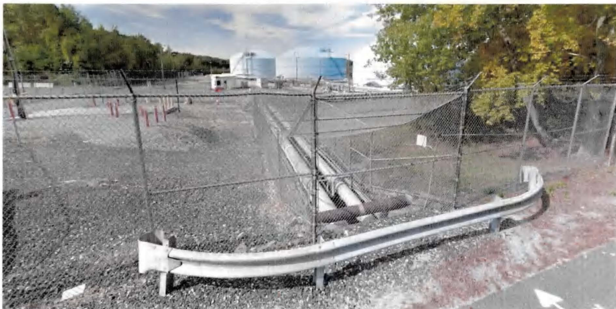
View of pipe entering under-road culvert looking west from roadway
