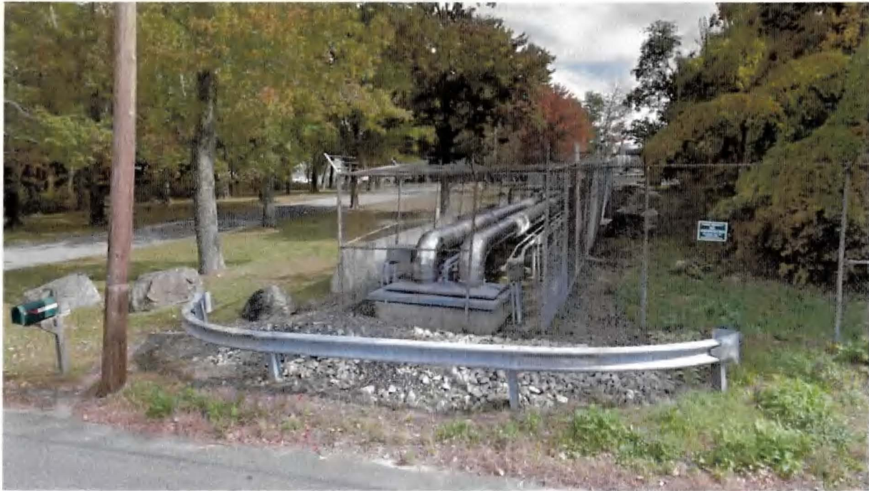
View of pipe entering under-road culvert looking east from roadway
