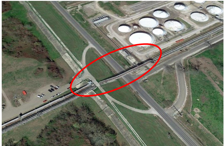
Figure 5: Transfer Pipeline to Barge Crossing Highway. Source: Google Earth
