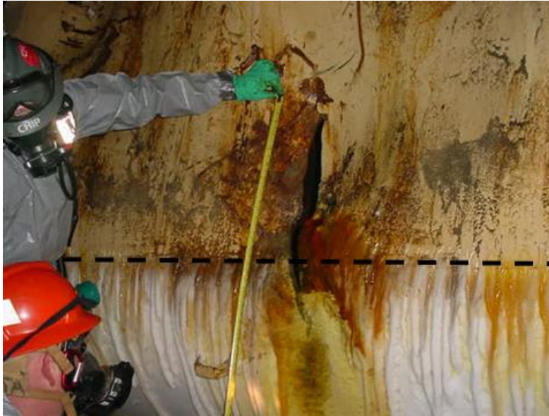
Figure 10: Rupture on Chlorine Tank Car. Source: Industrial Fire World, Green Cloud Rising
