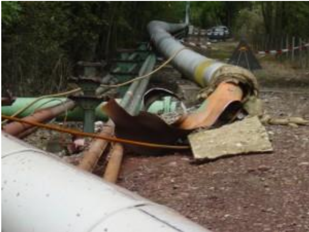
Figure 8: Ruptured pipeline. Source: DRIRE Rhône-Alpes
