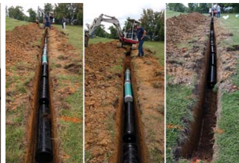
Figure 4. Pipe samples being buried.
