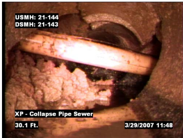
Fig. 1. Cross-bore of a natural gas distribution line in a sewer service lateral
