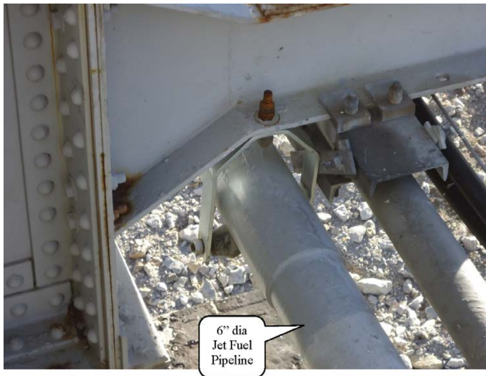
Pipe Roller Hanger Support at welded sleeve with a non-conductive roller. (Operator-provided photo)
