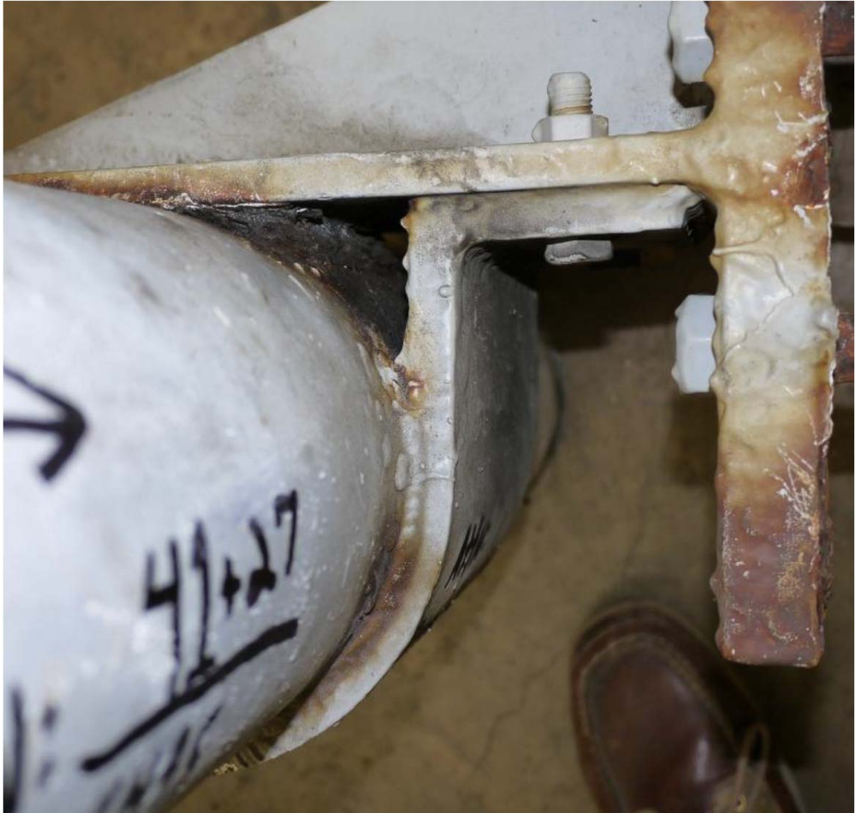
View of External Corrosion on Pipe/Support Assembly
