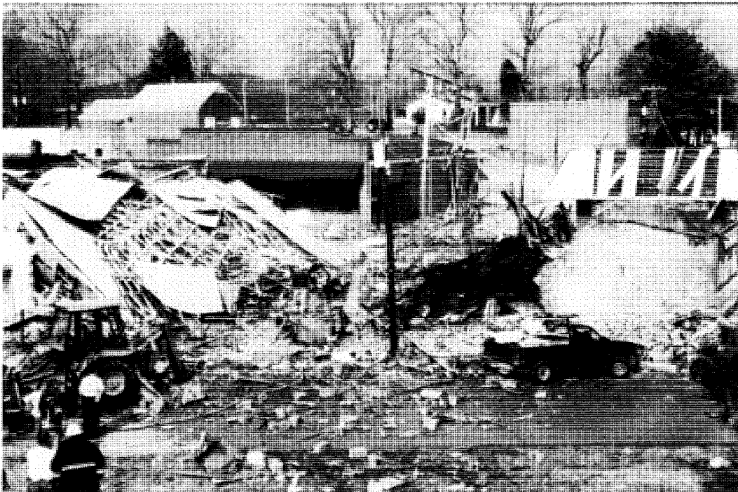
Figure 2. Damage to 404, 406, and 408 Alabama Avenue
