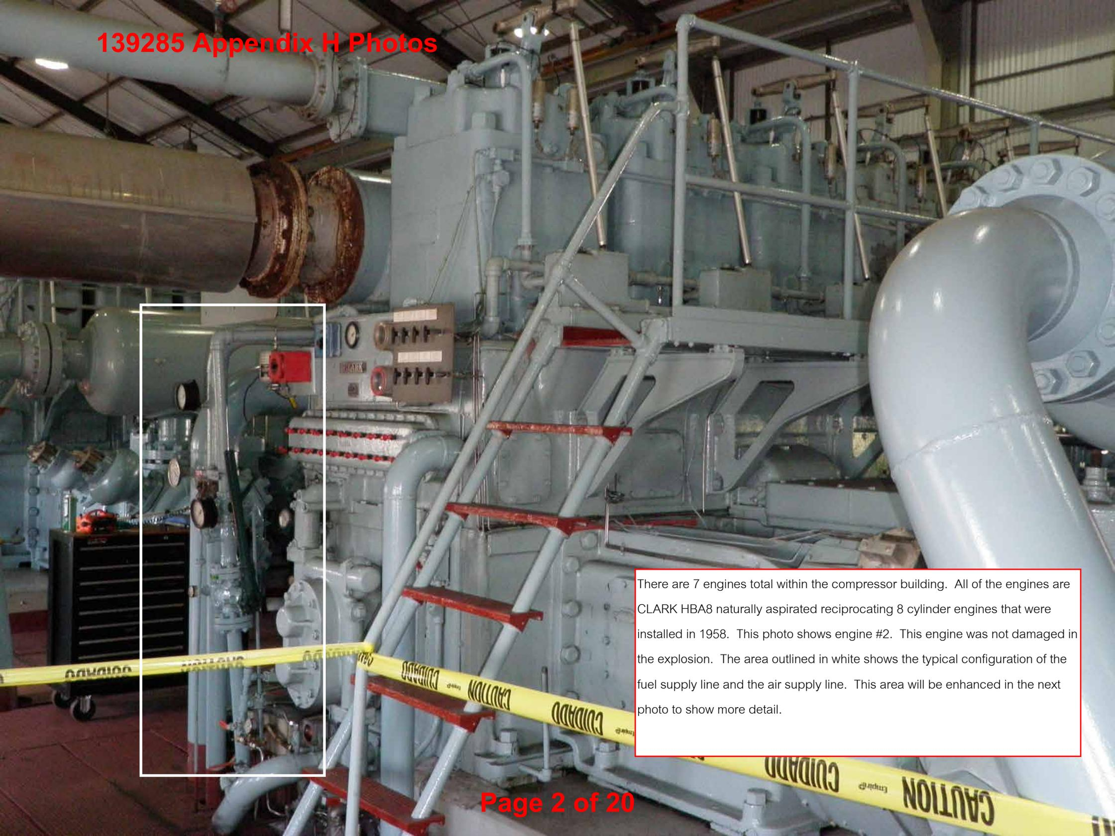
There are 7 engines total within the compressor building. All of the engines are CLARK HBA8 naturally aspirated reciprocating 8 cylinder engines that were installed in 1958. This photo shows engine #2. This engine was not damaged in the explosion. The area outlined in white shows the typical configuration of the fuel supply line and the air supply line. This area will be enhanced in the next photo to show more detail.
