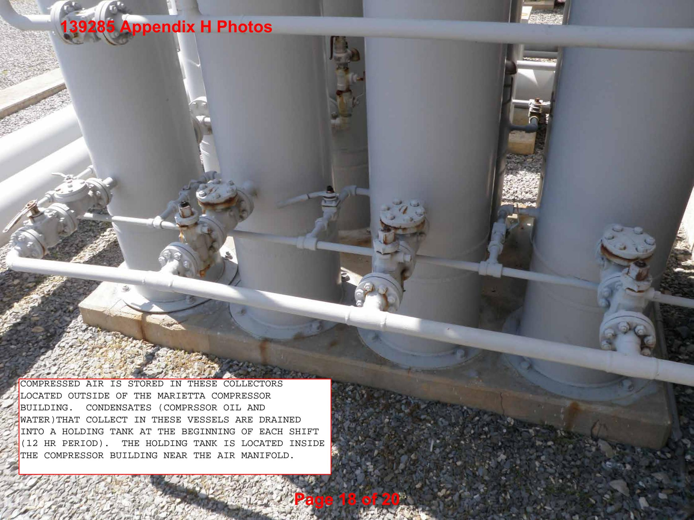
COMPRESSED AIR IS STORED IN THESE COLLECTORS LOCATED OUTSIDE OF THE MARIETTA COMPRESSOR BUILDING. CONDENSATES (COMPRESSOR OIL AND WATER) THAT COLLECT IN THESE VESSELS ARE DRAINED INTO A HOLDING TANK AT THE BEGINNING OF EACH SHIFT (12 HR PERIOD). THE HOLDING TANK IS LOCATED INSIDE THE COMPRESSOR BUILDING NEAR THE AIR MANIFOLD.
