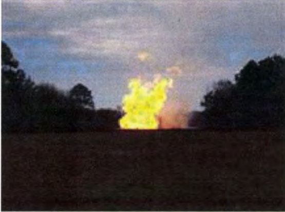
16-in South Main Pipeline after rupture and ignition
