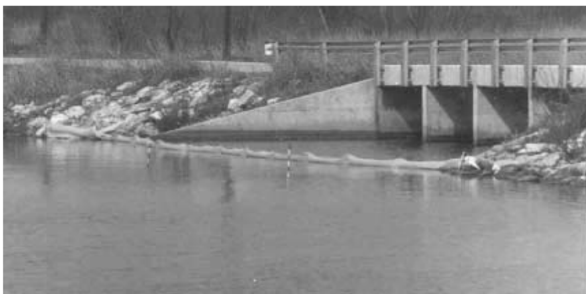
Figure 4-6. Exclusion booming of side stream.
