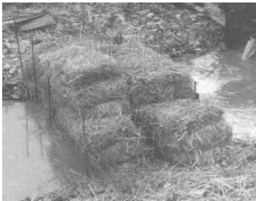
Figure 4-29. Hay filter barrier.
