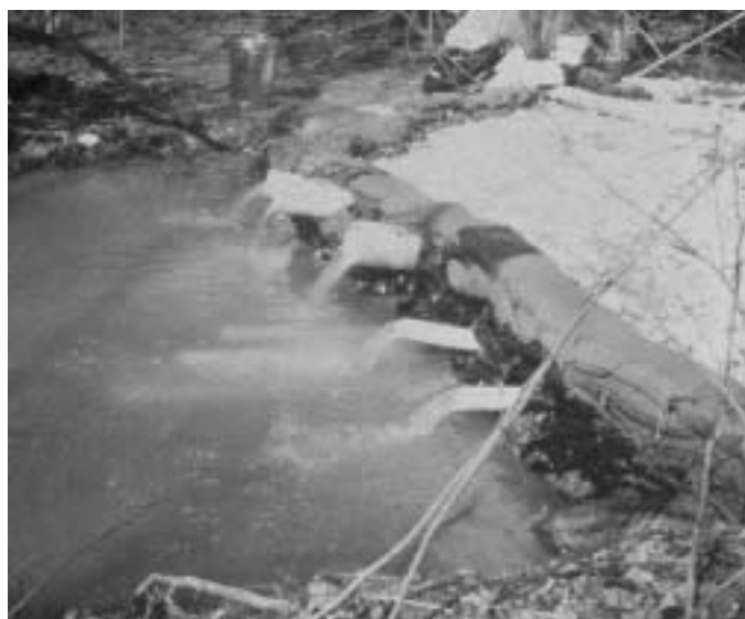
Figure 4-22. Sandbag underflow dam.
