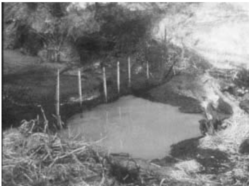
Figure 4-28. Sorbent barrier.
