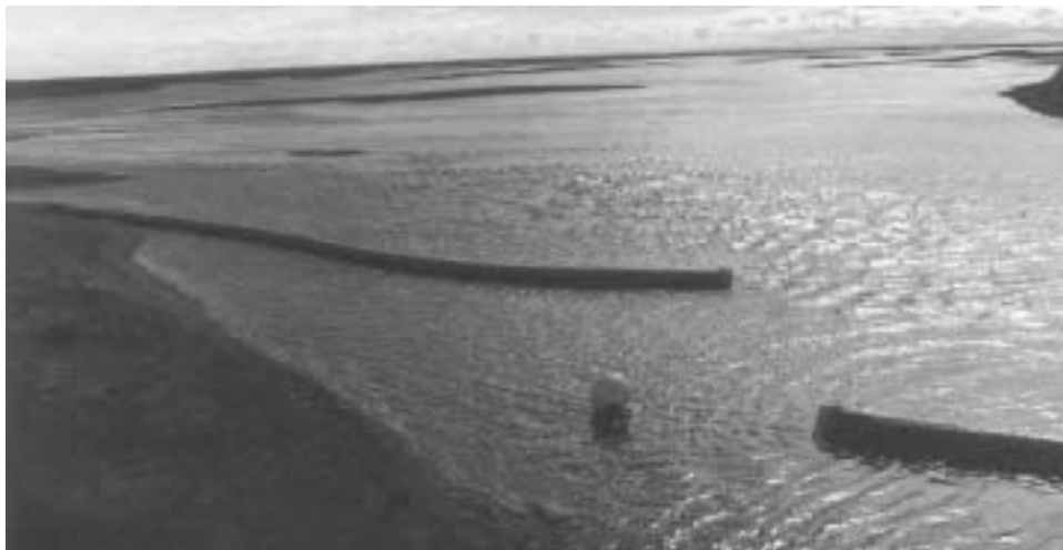
Figure 4-41. Cascade boom in inlet.
