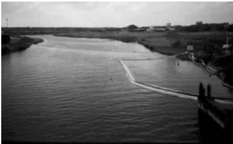
Figure 4-16. Boom at high tide.
