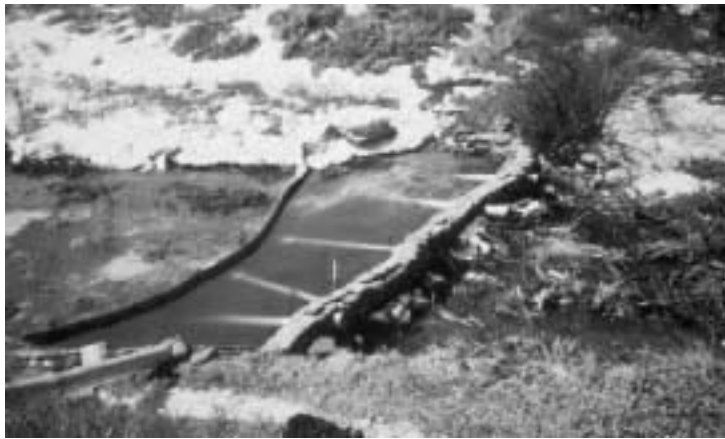
Figure 4-23. Underflow dam with debris boom.
