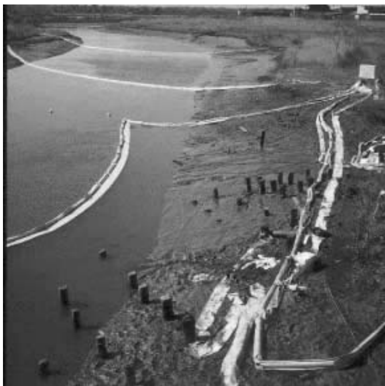
Figure 4-17. Boom at low tide.
