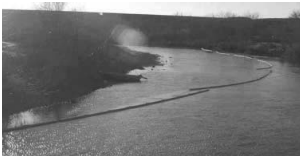
Figure 4-9. Cascade diversion booms deployed.
