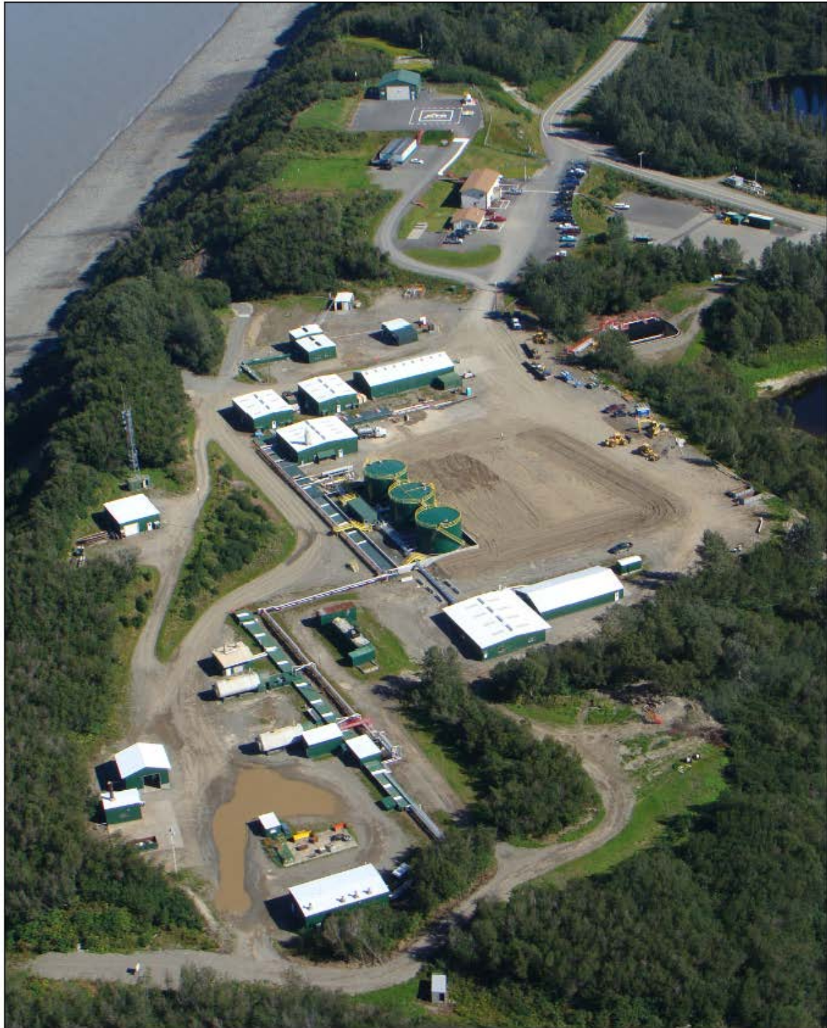
Figure I-4 XTO East Forelands “Onshore” Facility
