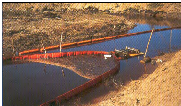
Figure D.2e Use of Booms with skimmer. Skimmer Operation Guidelines
