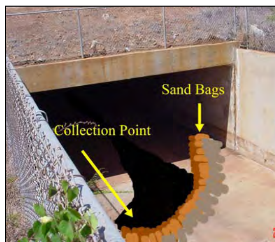
Figure C10b Low Flow Containment Berm.
