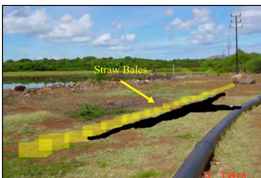
Figure C.6d Straw Bale Filter Barrier
