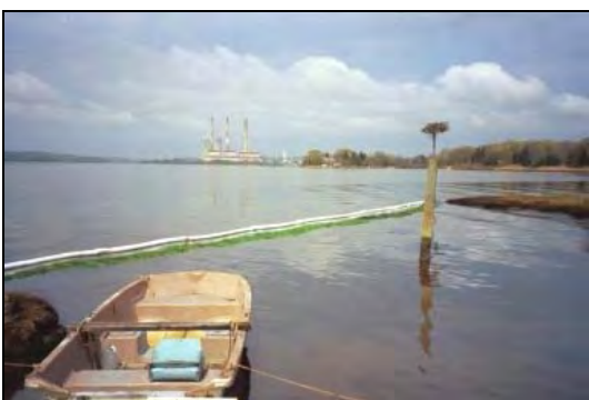
Figure C.5c Double Sorbent Booming
