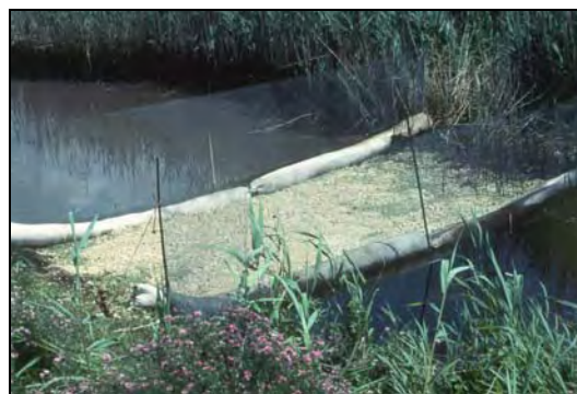
Figure C.6b Filter Fence – Tidal Flow
