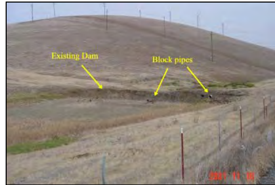
Figure C.8g Existing Control Structure.
