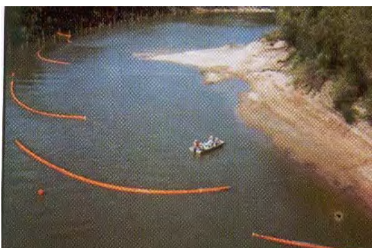
Figure C-3d. Cascade Booms in High Current
