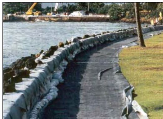
Figure C.5d Shoreline and Backshore Protection
