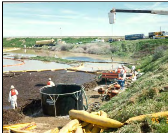
Figure D.1d Debris Management / Vacuum Recovery
