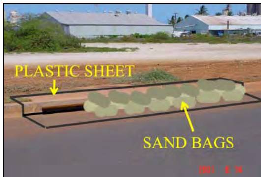
Figure C.9c Storm Drain Blocking
