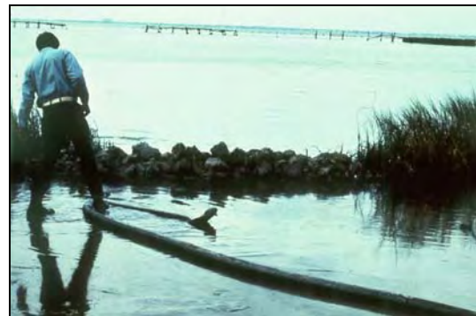
Figure C.7c. Earth Berm Across Wetland Channel
