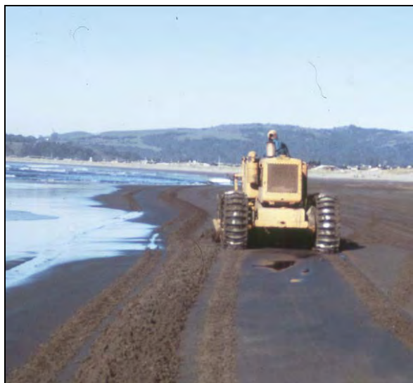
Figure D.4b Windrow Side Casting Using a Motor Grader
