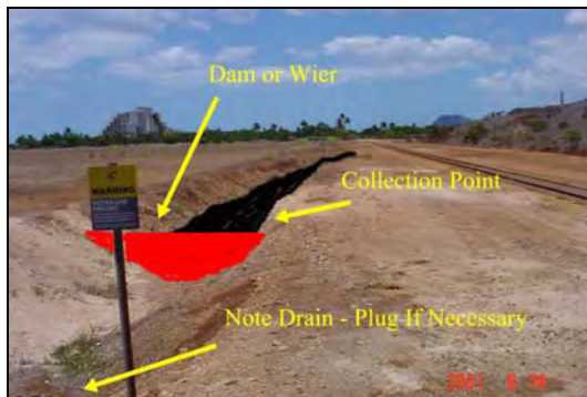
Figure C.7d Drainage Ditch Dam
