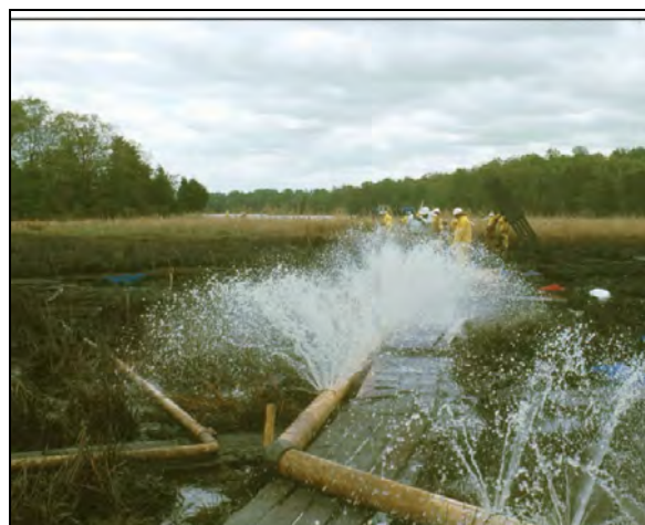
Figure D.6a Wetland Flooding Operation
