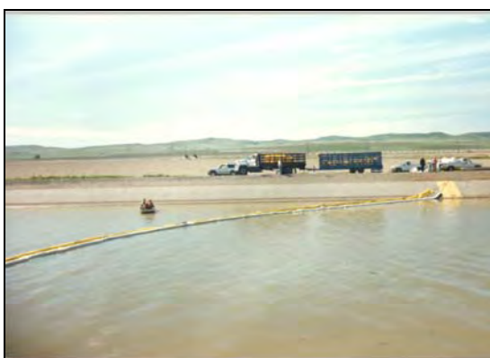
Figure C.10a Booming of Water Supply Canal (Courtesy Clean Bay Inc.)
