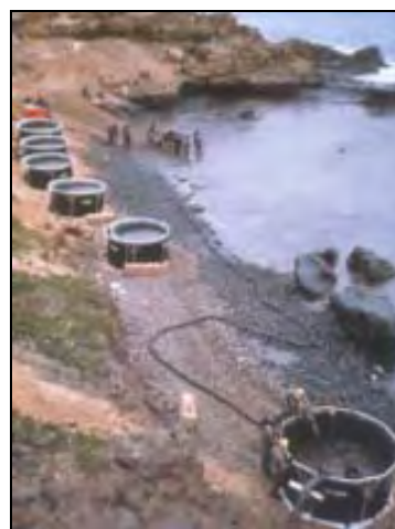
Figure C.2o Portable Storage Tanks
