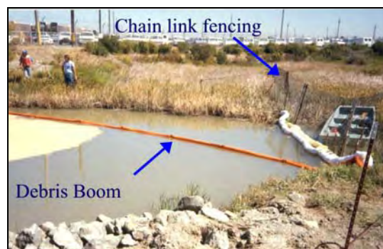
Figure C.6a Filter Fence – One Direction of Flow
