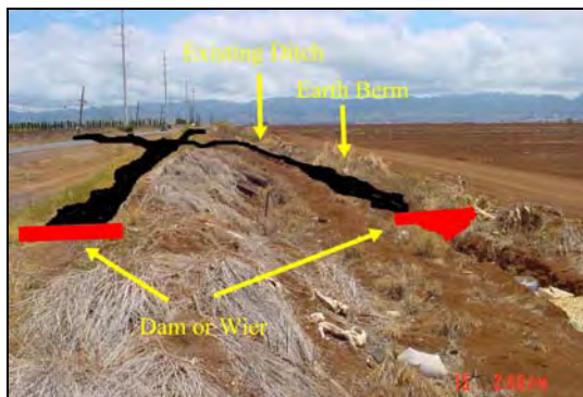
Figure C.7e Damming of Road Drainage and Irrigation Canal.
