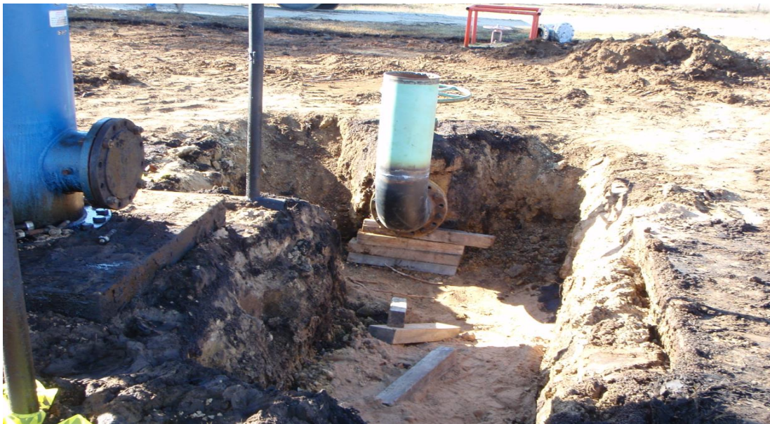
Figure 2 Strainer Site with start of replacement piping
