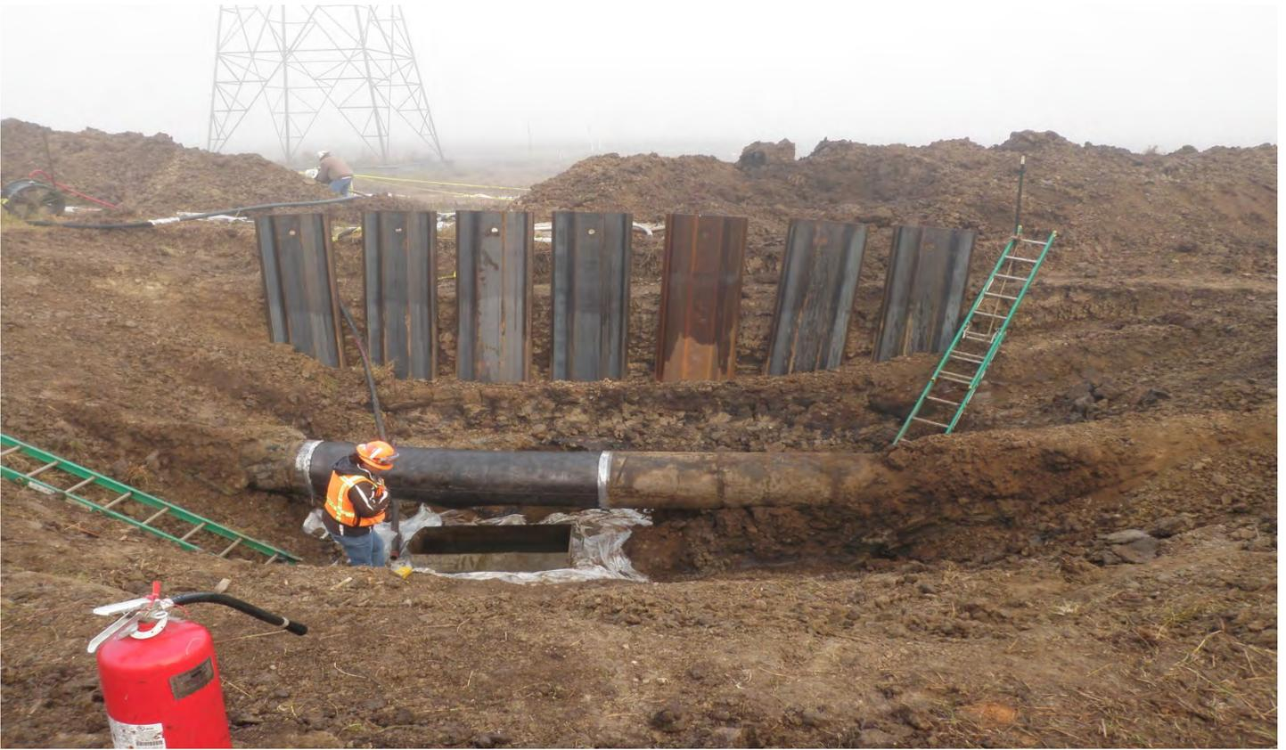
Shell Ho-Ho Pipeline Shoring for Repair of Pipeline 11-19-2010 8:2pAM
