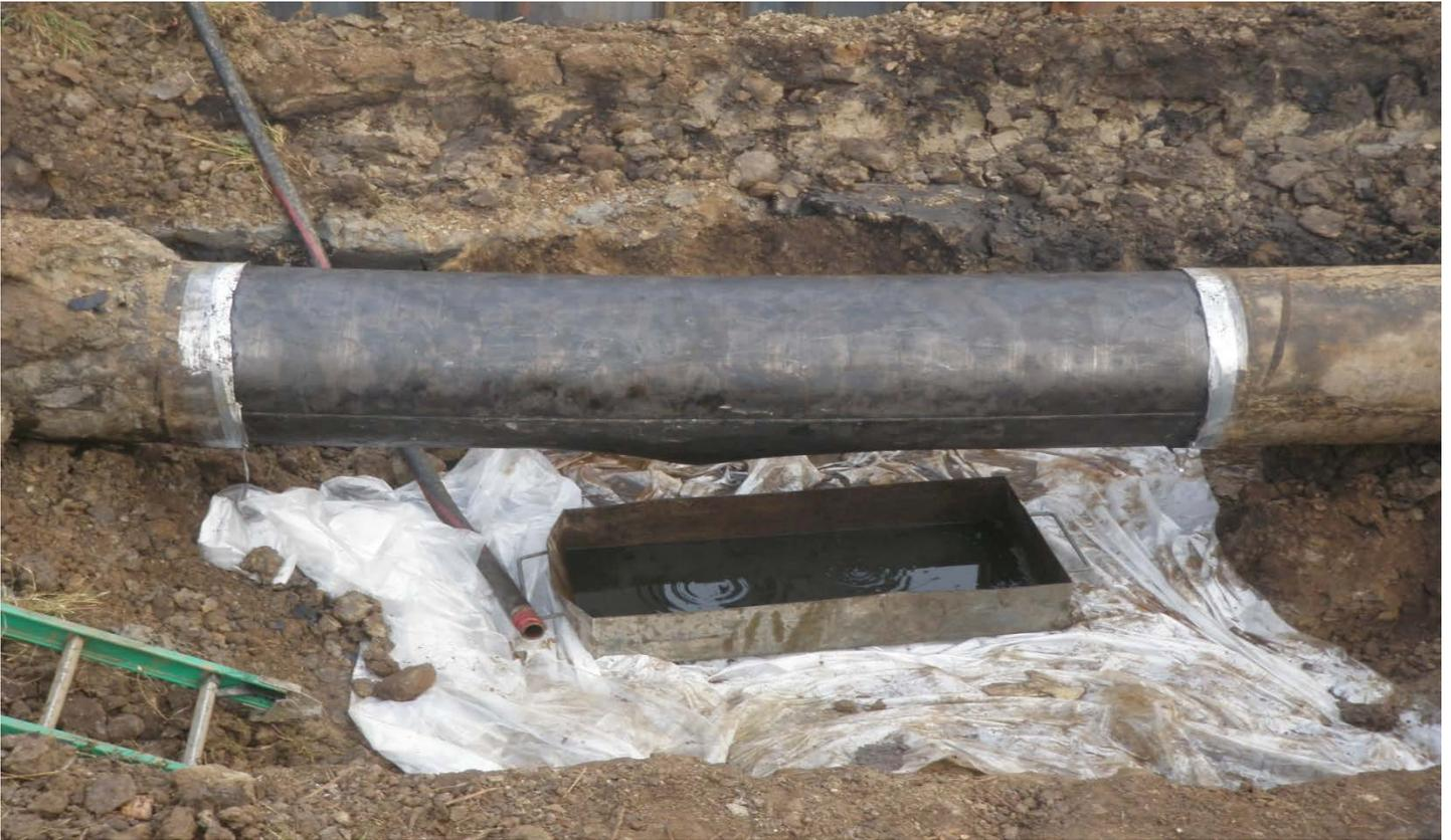
Shell Ho-Ho Pipeline Preparation of Segment for Cut-Out 11-19-2010 8:34AM
