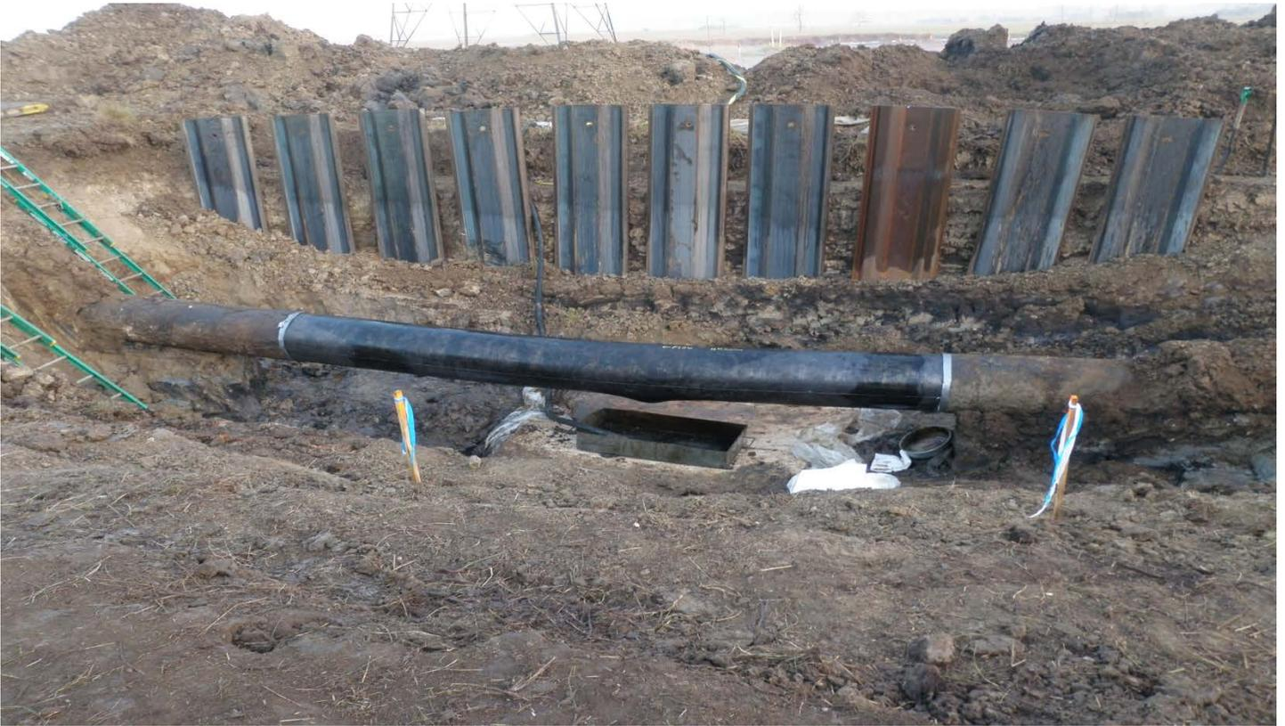
Shell Ho-Ho Pipeline Preparation of Segment for Cut-Out 11-20-2010 8:04AM
