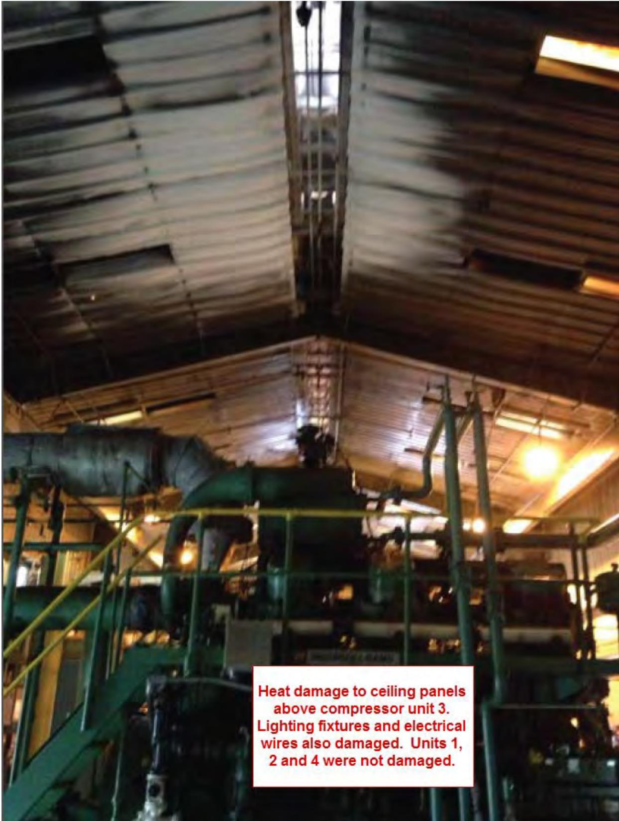
Heat damage to ceiling panels above compressor unit 3. Lighting fixtures and electrical wires also damaged. Units 1, 2 and 4 were not damaged.
