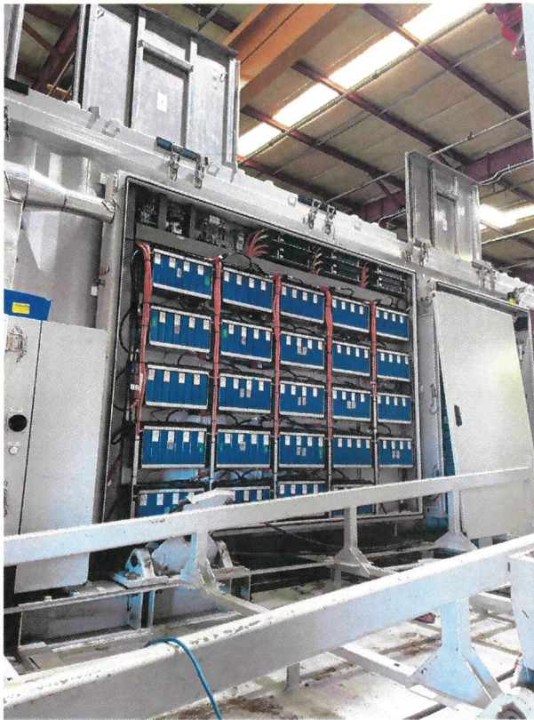
Exhibit Figure A-4. Interior views showing fixed battery modules, BMS equipment, high-voltage cabling, and structural/electrical modifications permanently dedicated to LT1200 functions.
