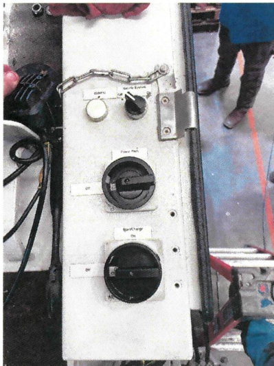
Exhibit Figure A-5. Representative LT1200 power/isolation controls and electrical protective components integrated into the LT1200 system.
