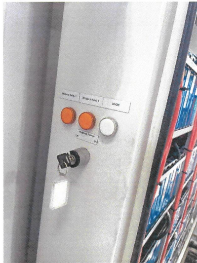
Exhibit Figure A-5. Representative LT1200 power/isolation controls and electrical protective components integrated into the LT1200 system.
