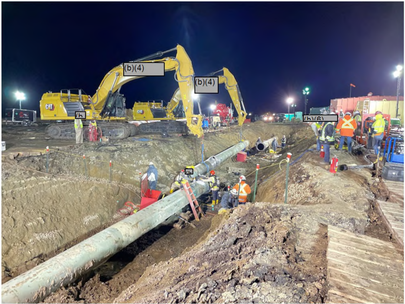
Figure 17. Cutout and removal of section of pipe with feature. PHMSA AID Photo.
