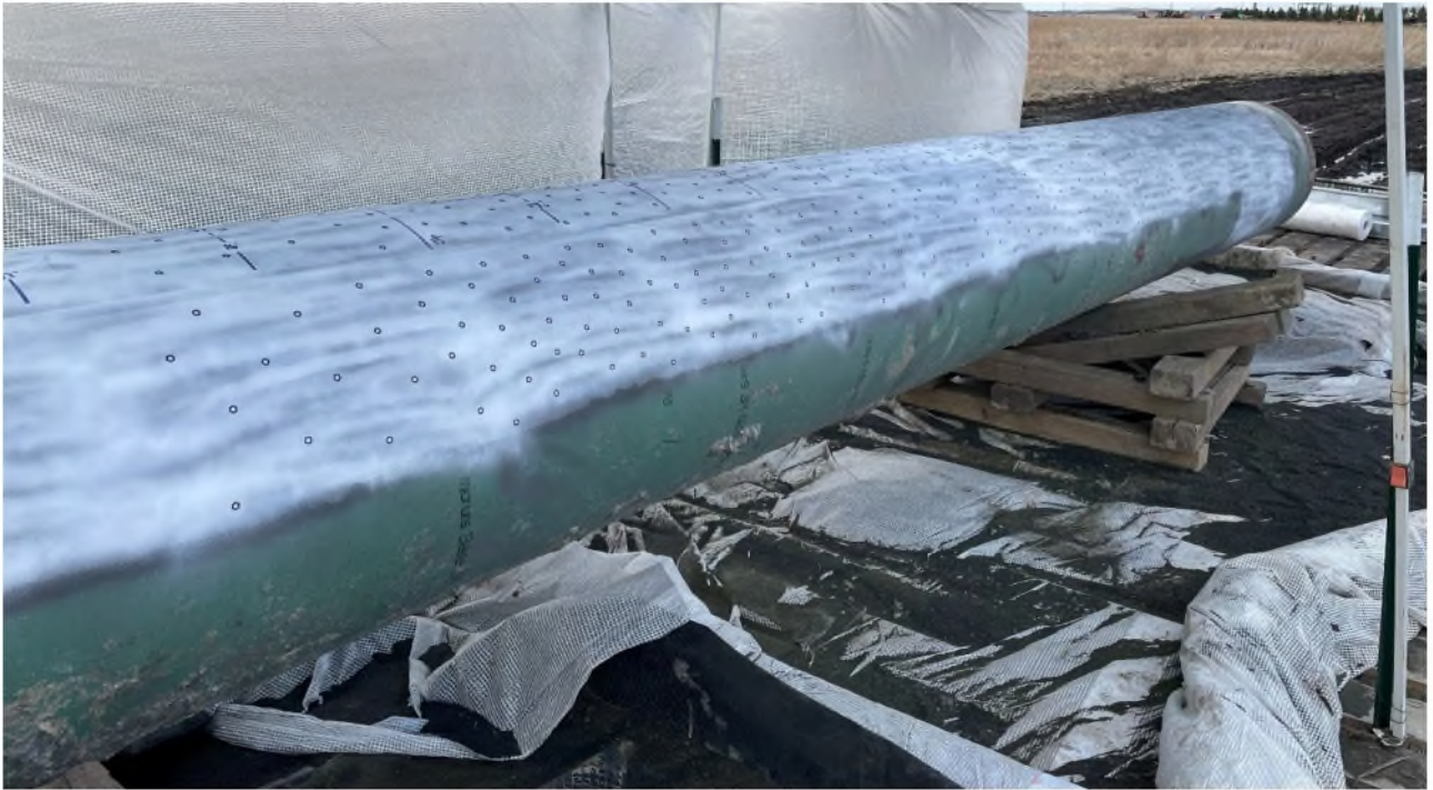
Figure 18. Segment with failure origin prepared for on-site non-destructive testing. PHMSA AID photo.
