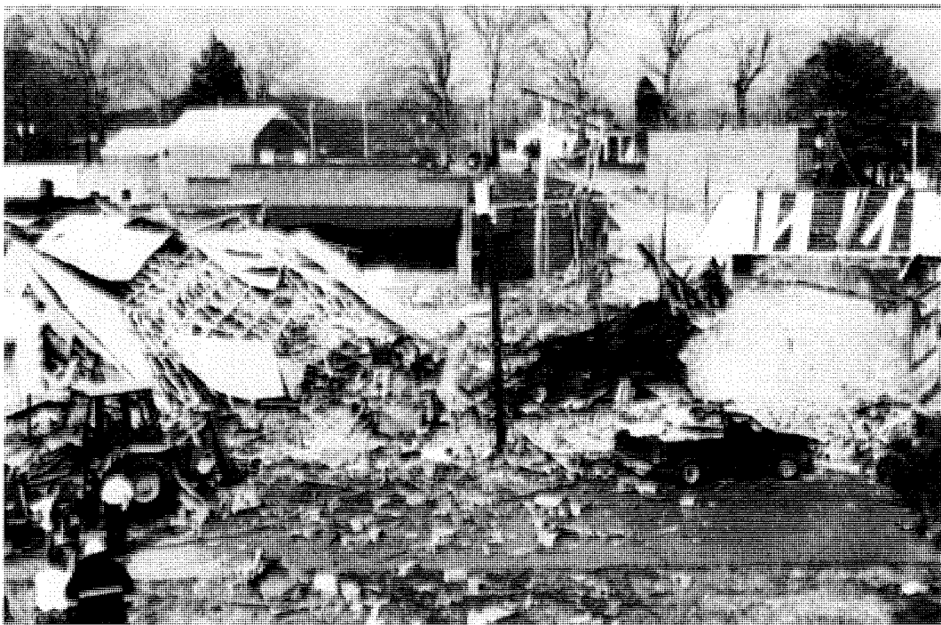
Figure 2. Damage to 404, 406, and 408 Alabama Avenue
