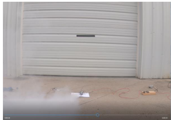
Picture 2: Stat-X 30E activated
