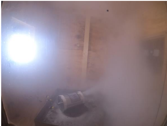
Picture 10: Stat-X 500E Smoke Box Activated
