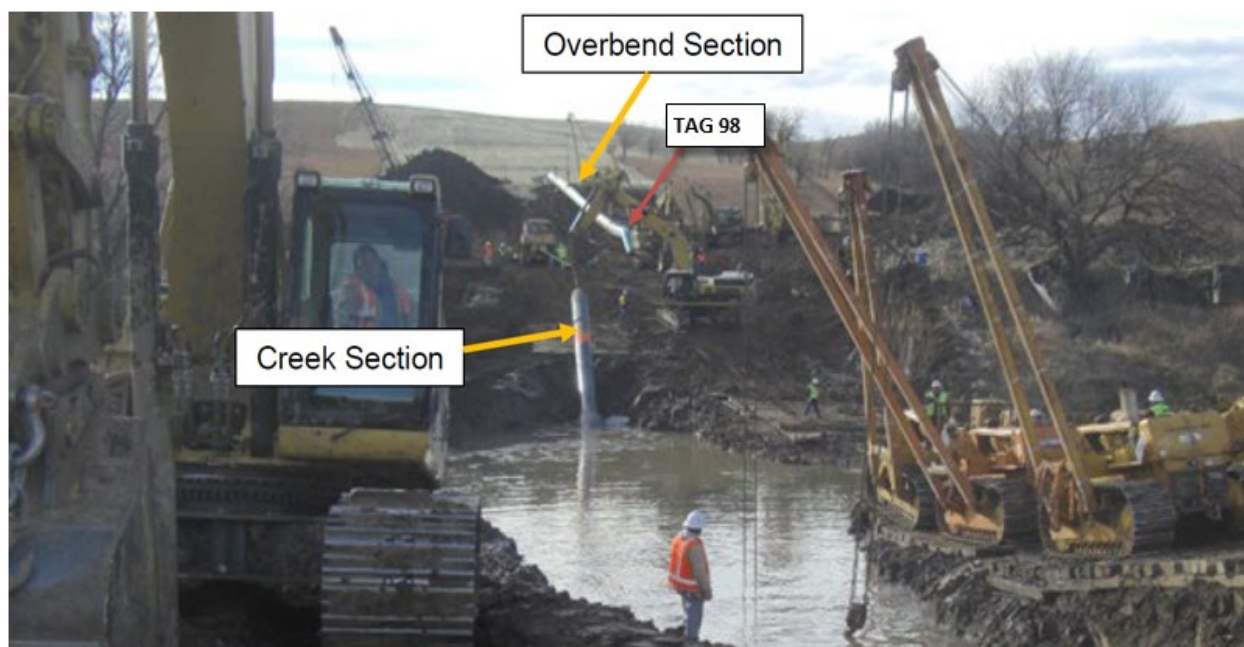
Figure 16. December 2010 WRP Work at the Failure Location Looking South in the Downstream Direction (TAG 98 Label Added by PHMSA), Photo from TC.
