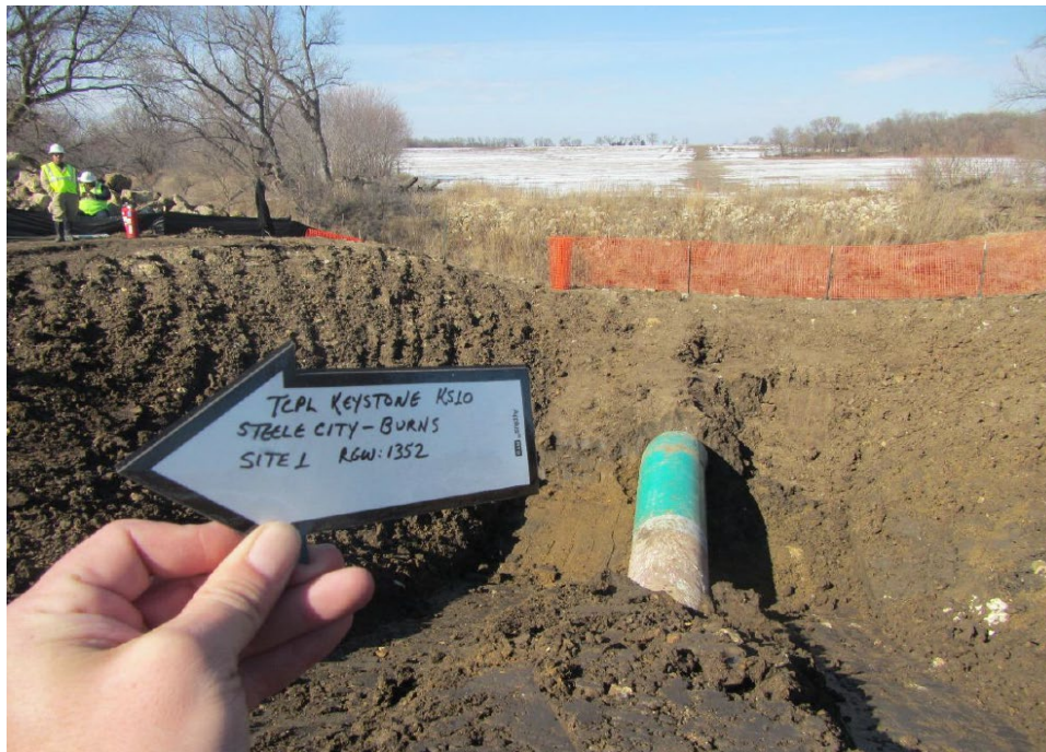
Figure 17. Photo of TAG 98 Fitting Assembly During the 2013 Ovality Inspection Showing the Extent of Excavation. The Excavation Did Not Add or Decrease Any Stress on the Pipeline, Photo from TC.
