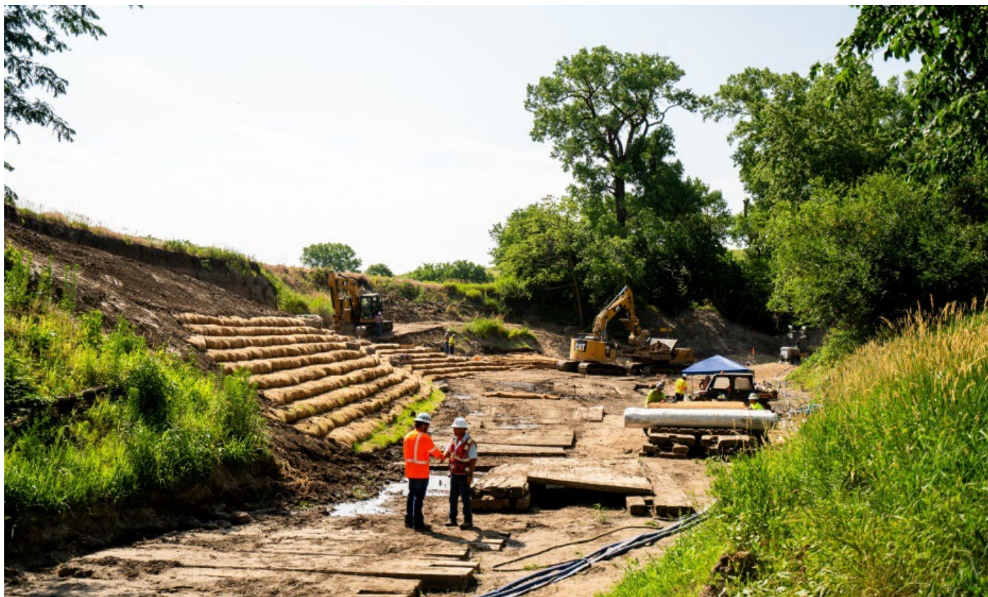
Figure 3. Keystone Cushing Extension Pipeline Crossing of Mill Creek Near the Failure. Dry Creek Bed and Clean-up After River Diversion (South is to the Left), Provided by TC.
