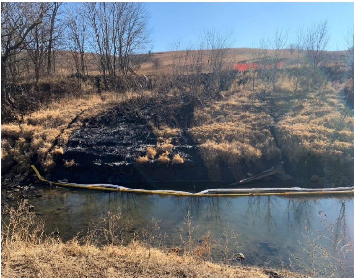
Figure 6. South Creek Bank Showing Shallow Soil Slippage, Pipeline Runs from Creek Uphill to Orange Fencing.
