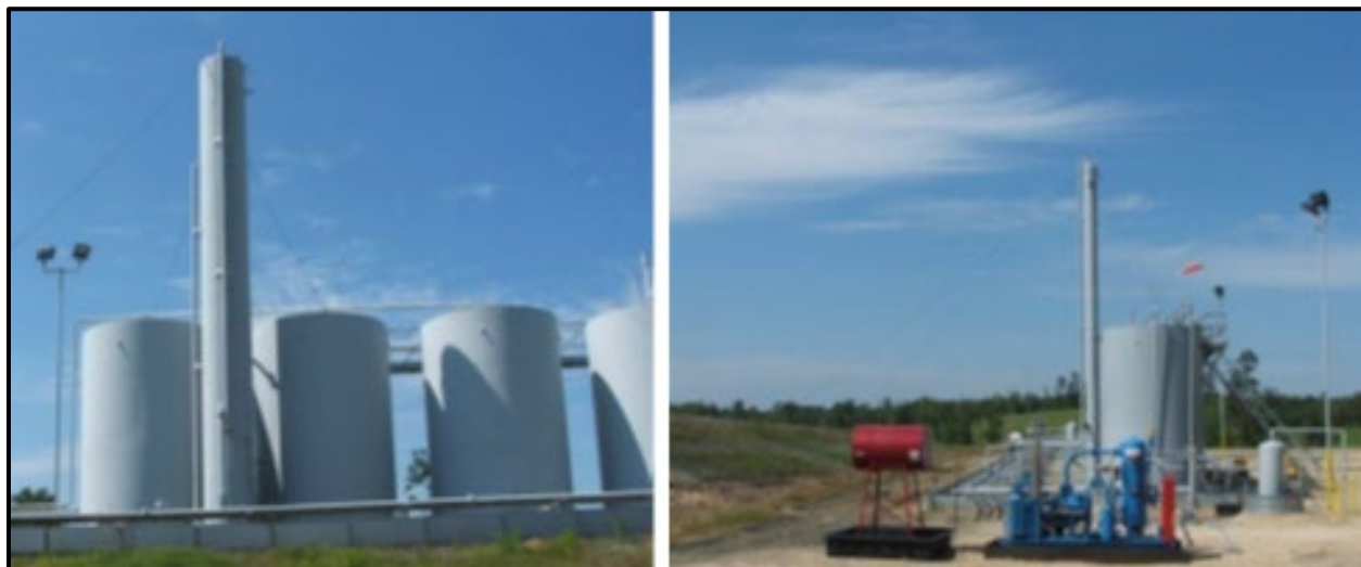
Figure 27: Typical Tank Battery VRT (Left) and VRU (Right) (Courtesy of Hy-Bon Engineering Inc.)
