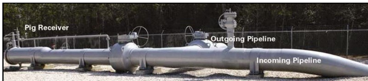
Figure 26: Example Pig Receiver on a Natural Gas Transmission Pipeline (Courtesy of Metropolitan Engineering, Consulting & Environmental Services)
