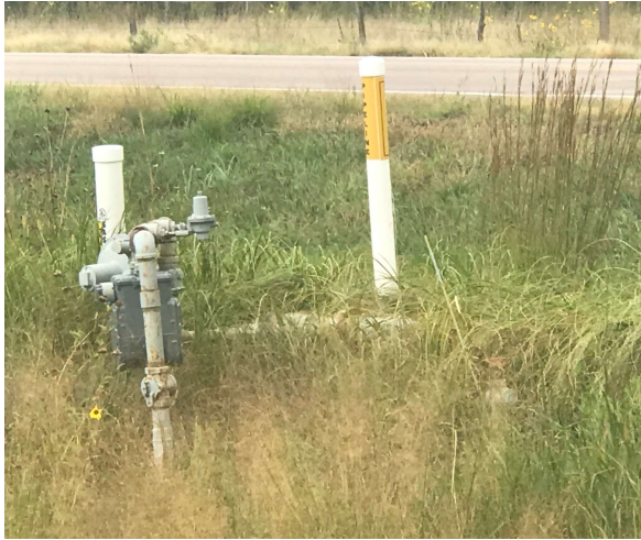
Existing above-ground 4" steel vaguely visible in front of marker post to be replaced with 4" HDPE pipe and 4" valve.
