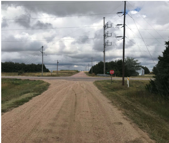
General view looking north on 500 Avenue. Existing 4" steel crossing Hwy 108 diagonally to marker post east of power switch pole on north side. 2" HDPE to be inserted through existing 4" steel under Hwy 108.
