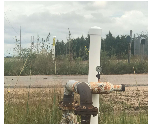
4" steel pipe crossing 498 Avenue to be replaced with 4" HDPE. Existing 3 and 4" valves and above-ground piping to be replaced with 4" valve and 2" riser for pressure test station.
