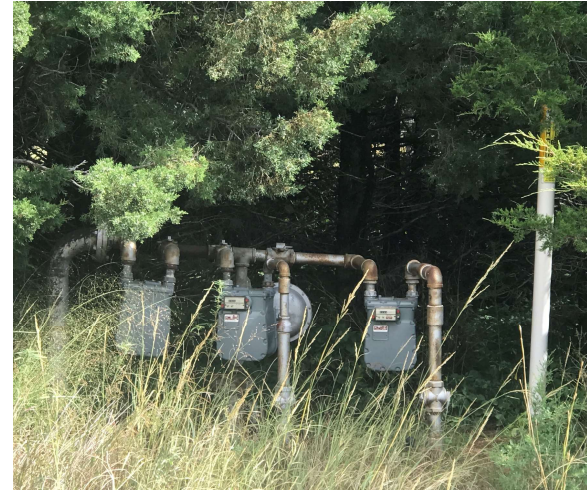
Existing 4" steel behind center meter to be replaced with 2" HDPE riser at this location. Two service lines to be connected to new 2" HDPE main line riser.
