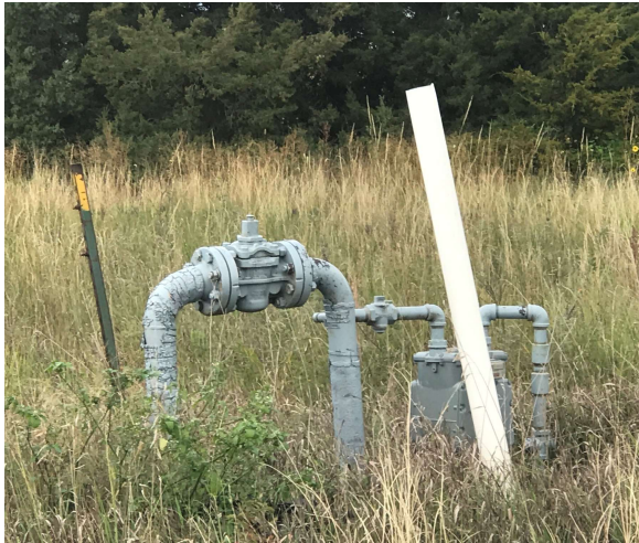
Existing 3" steel firebreak to be replaced with 2" HDPE riser to feed meter shown.
