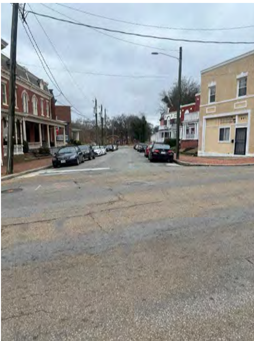
North on N 21st St. Single family homes on either side of roadway.
