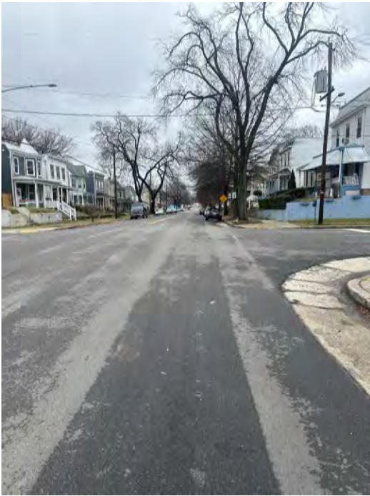
Venable St. and N21st St. intersection.
