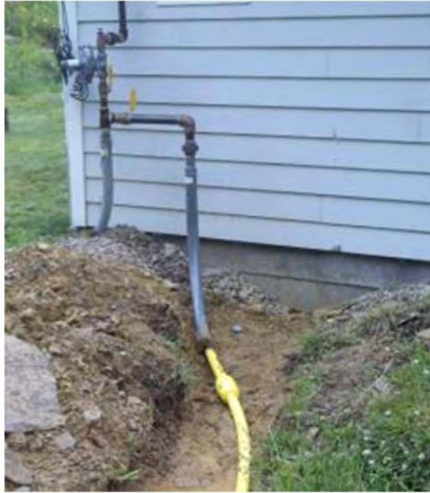
Photo 1. Representative photo showing new PE service line connection to residential meter.
