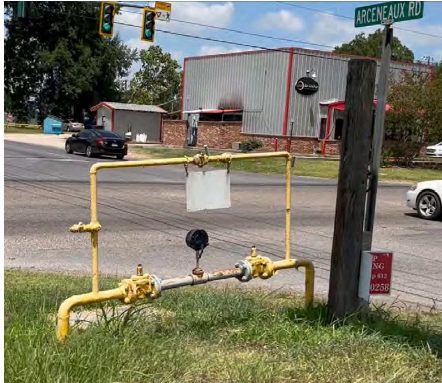
Photo 3. Representative photo showing regulator station within the APE.
