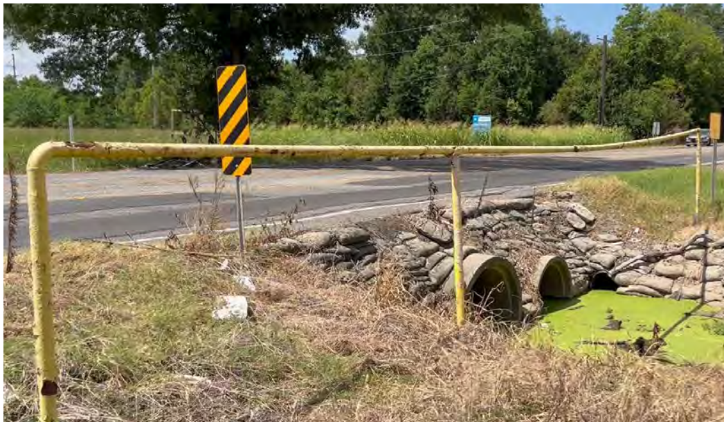
Photo 4. Representative photo showing exposed piping over a water (coulee) crossing within the APE.
