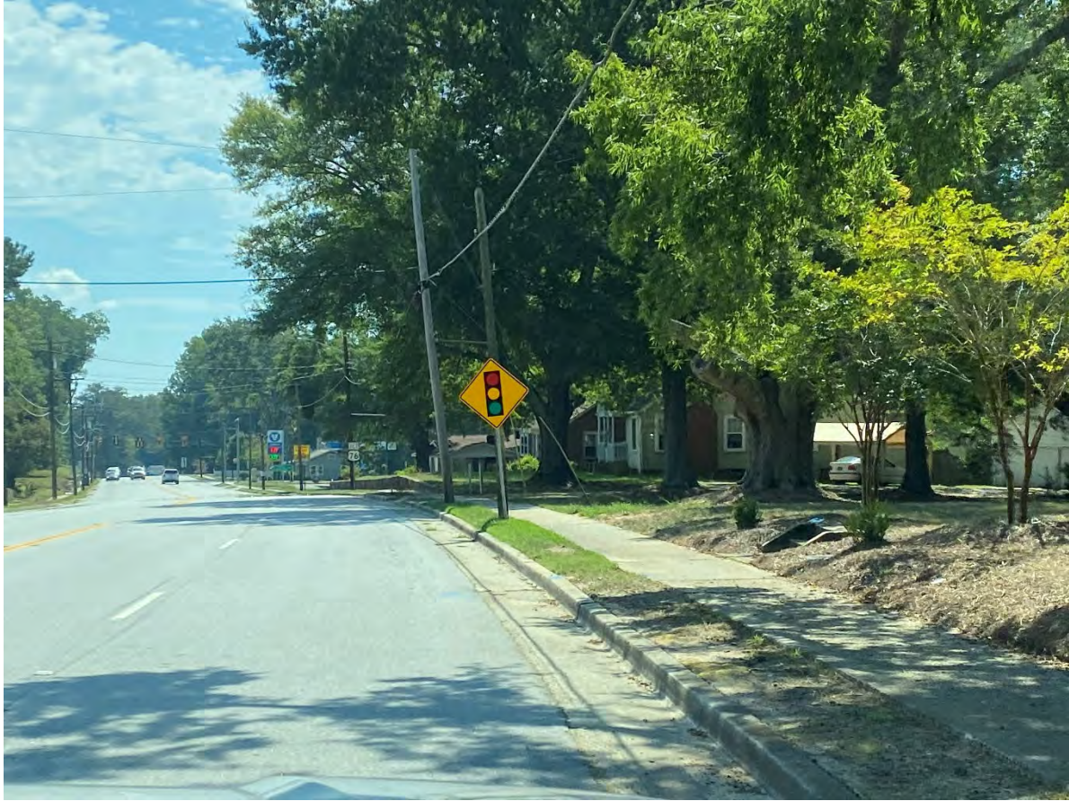
Typical right-of-way for the Laurens pipeline replacement project along West Main Street (Hwy 76) in Laurens, SC. The proposed pipeline will be installed approximately 5-10 feet from the right side of the street. This photo was provided to show existing sidewalk and powerlines co-located with the existing natural gas pipeline. This photo was taking facing east, showing the southern side of West Main Street. This photo was taken just northwest of the Valero located at 529 Church St in Laurens, SC.
