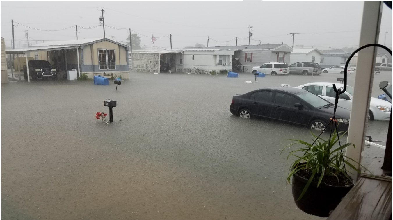
Figure 2-36: Flooding impacting Bayou Vista
