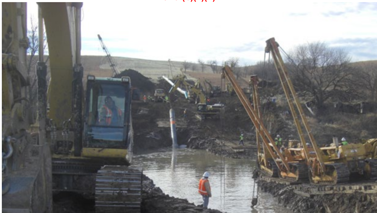
Figure D.19. Use of Sidebooms During Replacement of TAG 98 (December 10, 2010)
