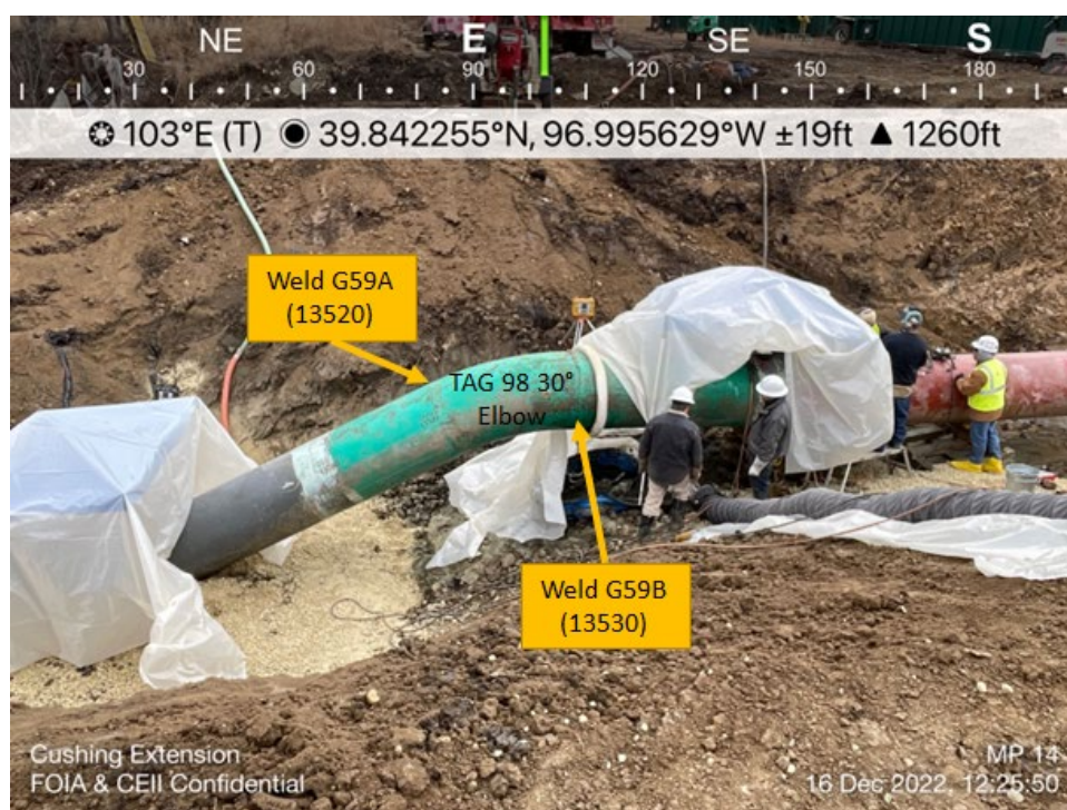
Figure 8. Excavated Bend Assembly – December 16, 2022
