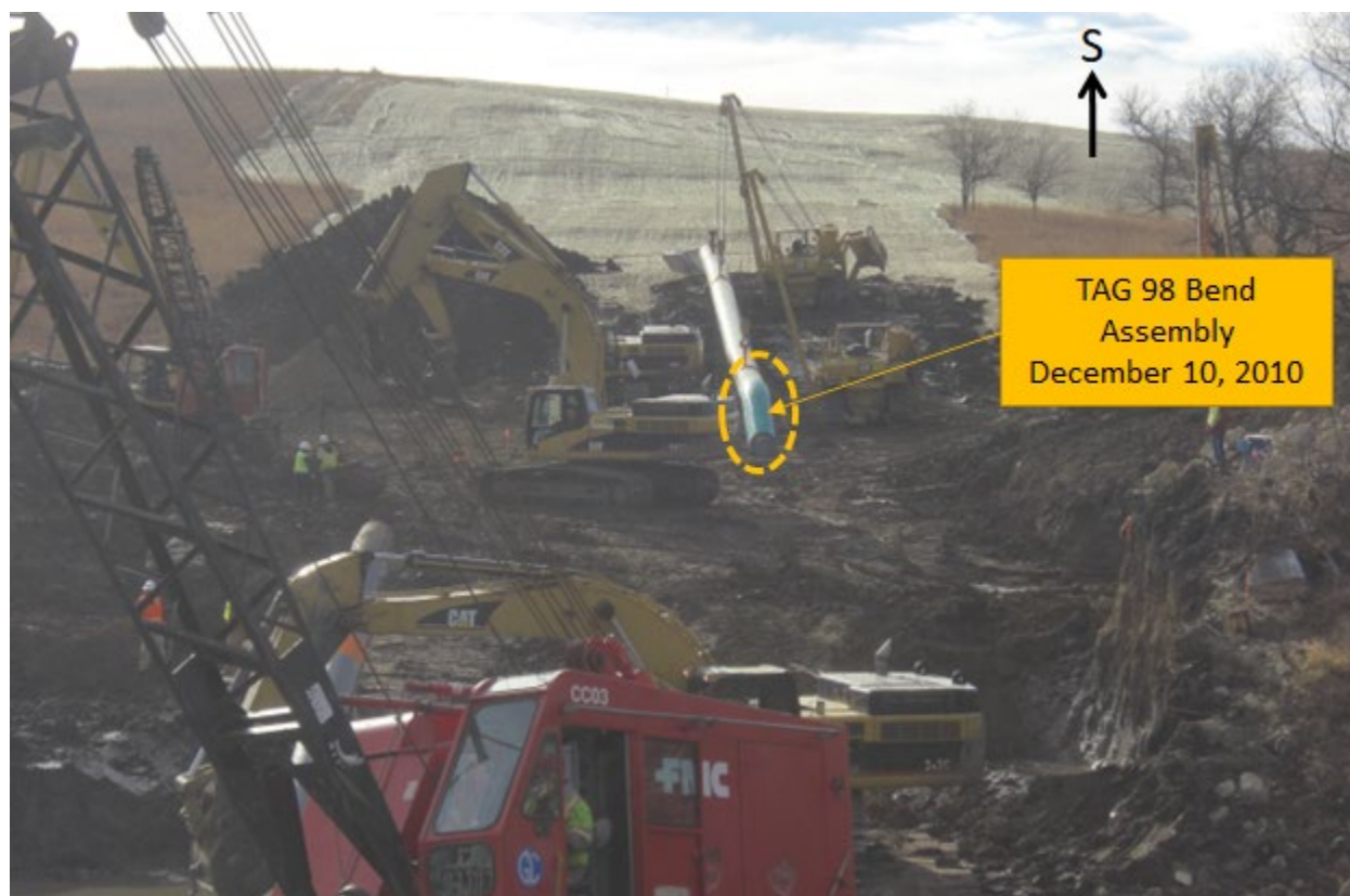
Figure 10. TAG 98 Bend Assembly (BND 350) During Replacement (December 10, 2010)
