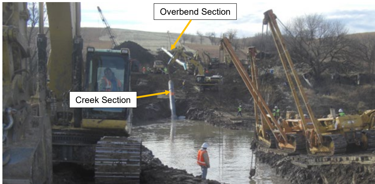
Figure 32. Use of Sidebooms During Replacement of TAG 98 (December 10, 2010)
