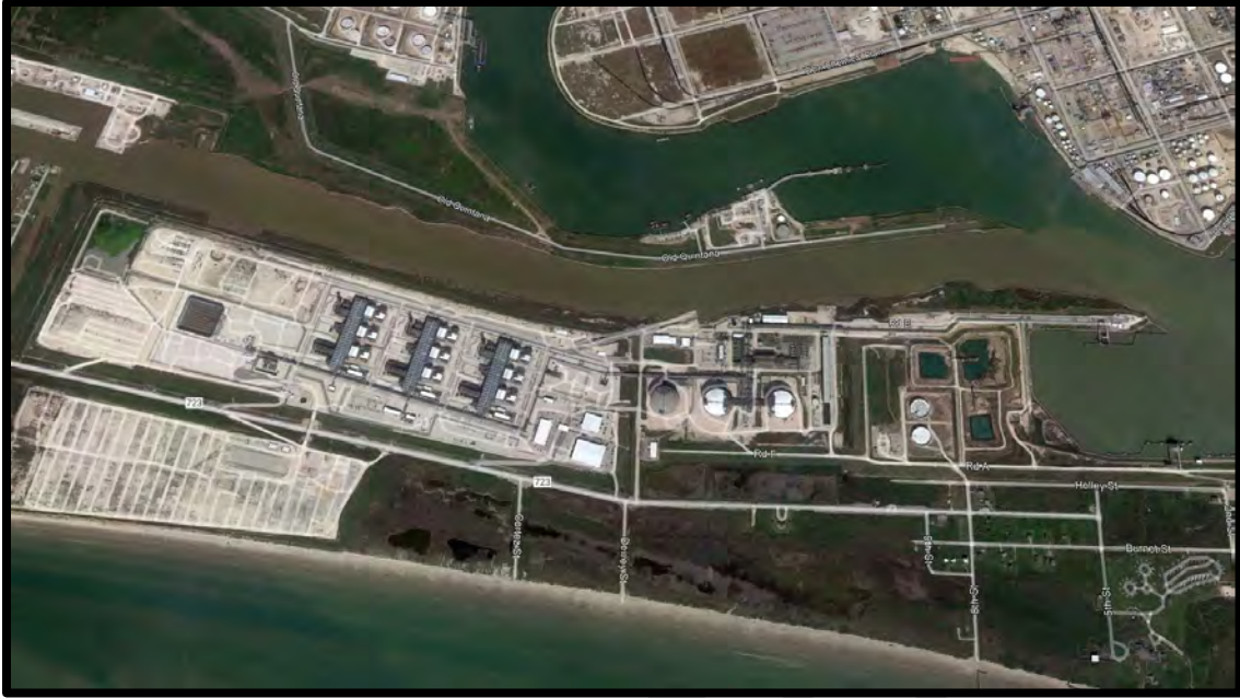
Figure 5 - Overhead View of Freeport LNG Facility – Quintana Island, Texas
