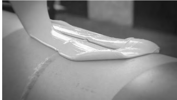
Pouring the coating onto the girth weld
