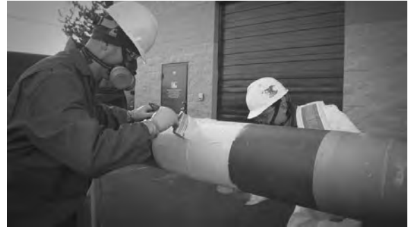
Brush around the weld bead to ensure adequate coating thickness to all high asperity areas.
