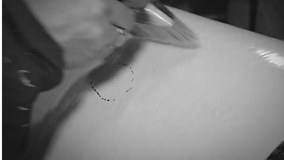
Wipe surface area clean with a brush.
