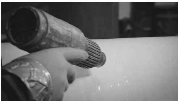
When preheating, DO NOT burn the existing coating.
