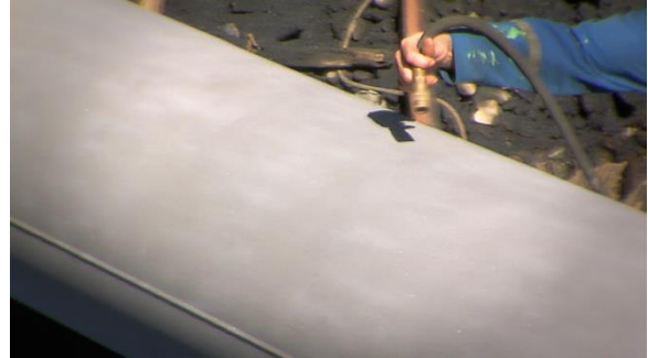
Or use dry compressed air to clean surface area.
