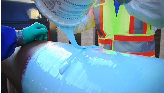
Apply the balance of the kit to the weld bead.
