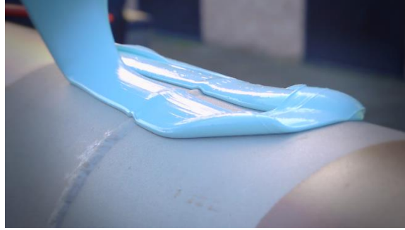
Pouring the coating onto the girth weld
