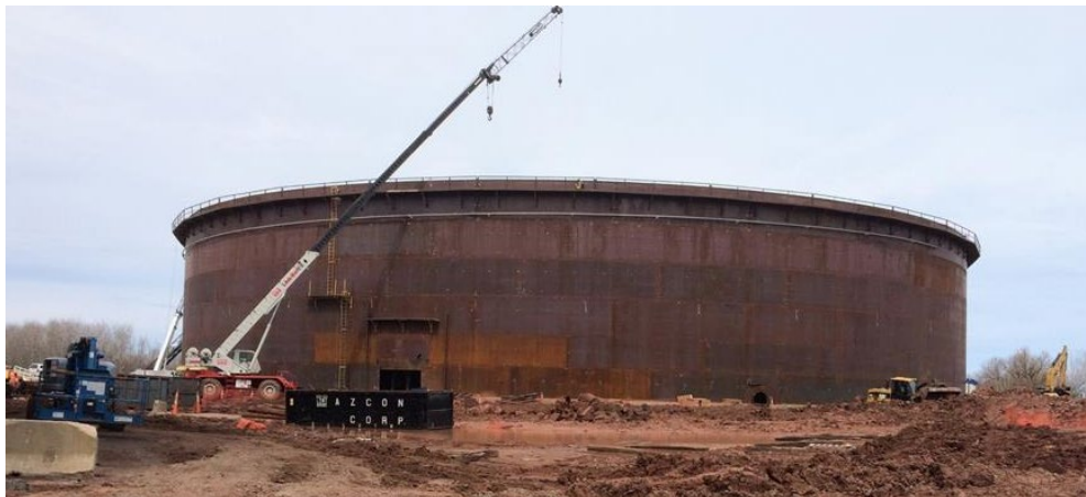
Figure 3 – API 650 Tank under construction (Photo courtesy of PHMSA)
