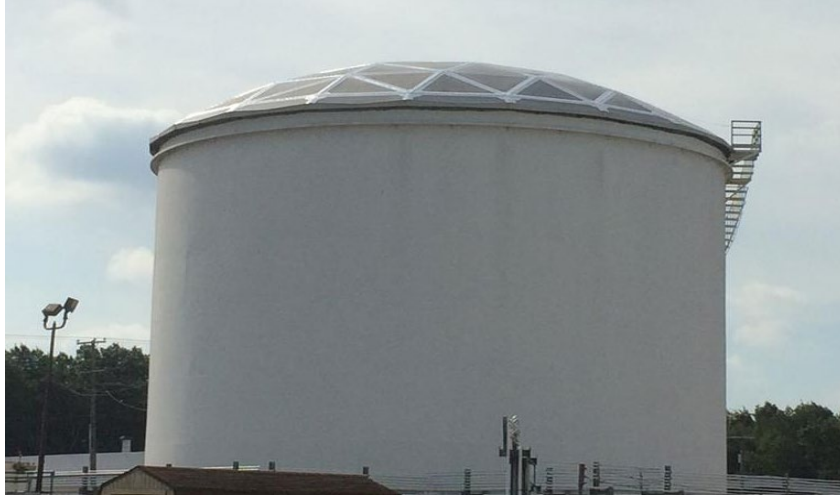
Figure 1 – API 650 Tank (Photo courtesy of PHMSA)
