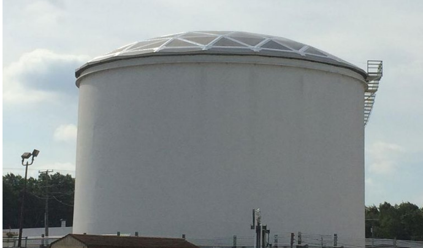
Figure 1 – API 650 Tank (Photo courtesy of PHMSA)
