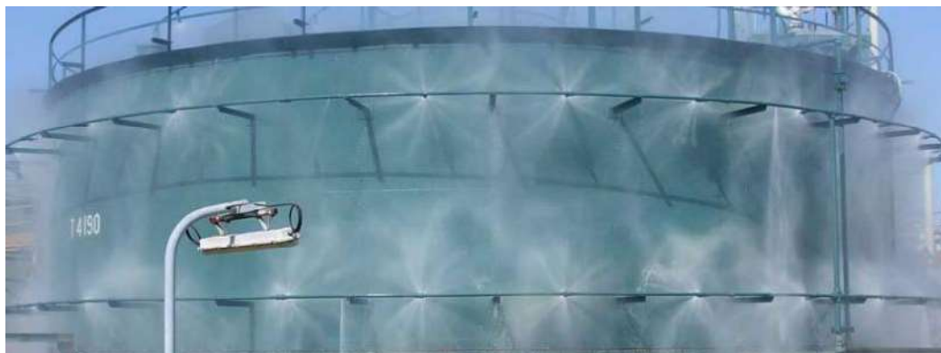
Figure 8 Evaluating various LNG safety measures such as water curtains to determine efficacy. Courtesy VFP Fire Systems.
