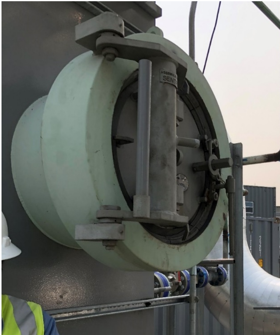
Figure 4. Photograph provided by AGT showing the closure on Filter Separator FS-01 that experienced a seal failure.
