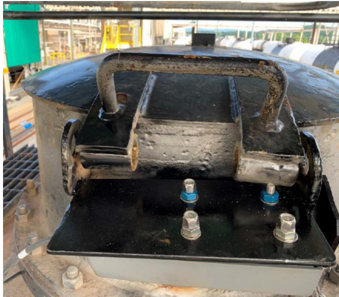
Figure 4.4 - Lock Mounting Plate
